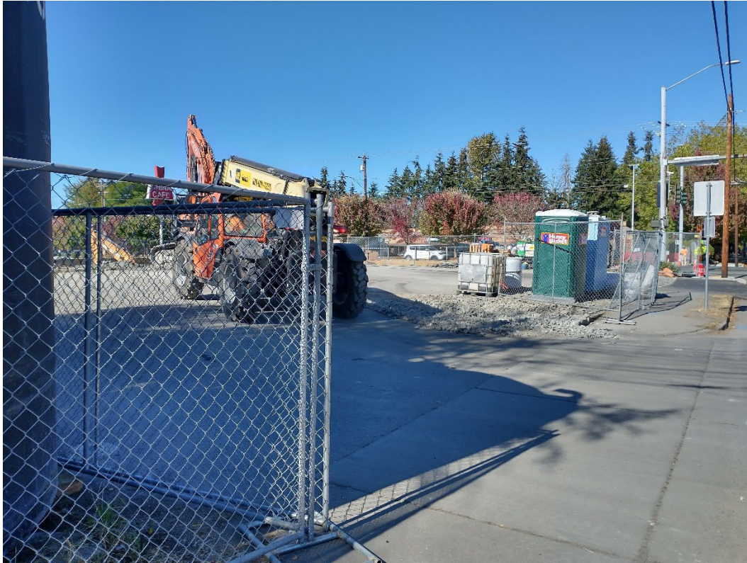
View from south site gate on 68 th Ave., facing northwest.
