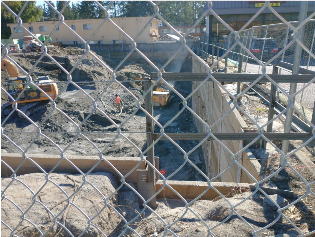
View of excavation and shoring wall from 196 th St, facing south.
