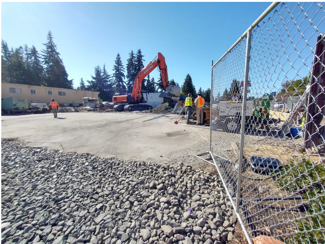
View from north site gate on 68 th Ave., facing southwest.
