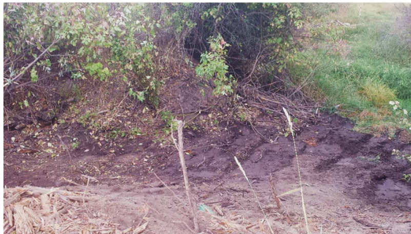
Debris removed from Wetland Debris Area 2 on September 24, 2015 (facing west-southwest).
