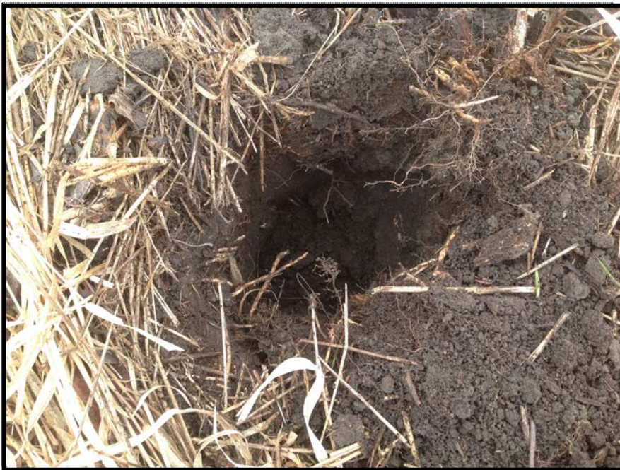
General view of SP-5 soil pit.
