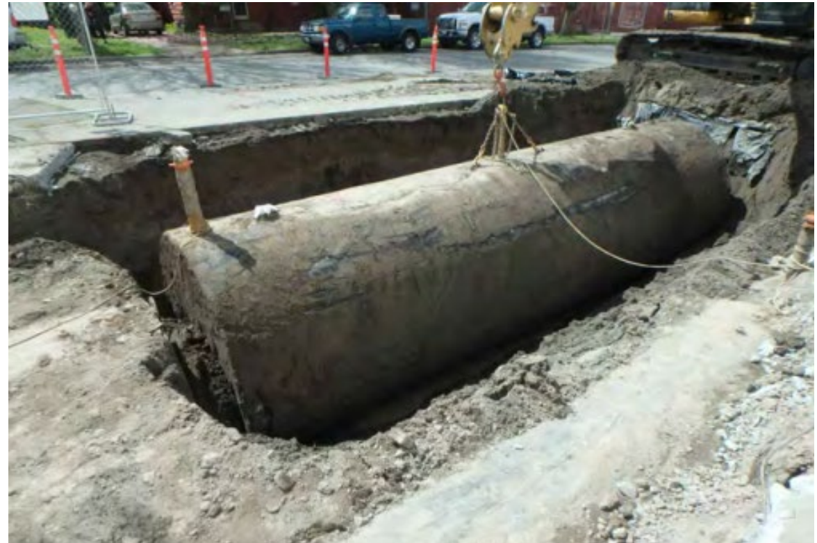
Underground storage tanks removed from the site
