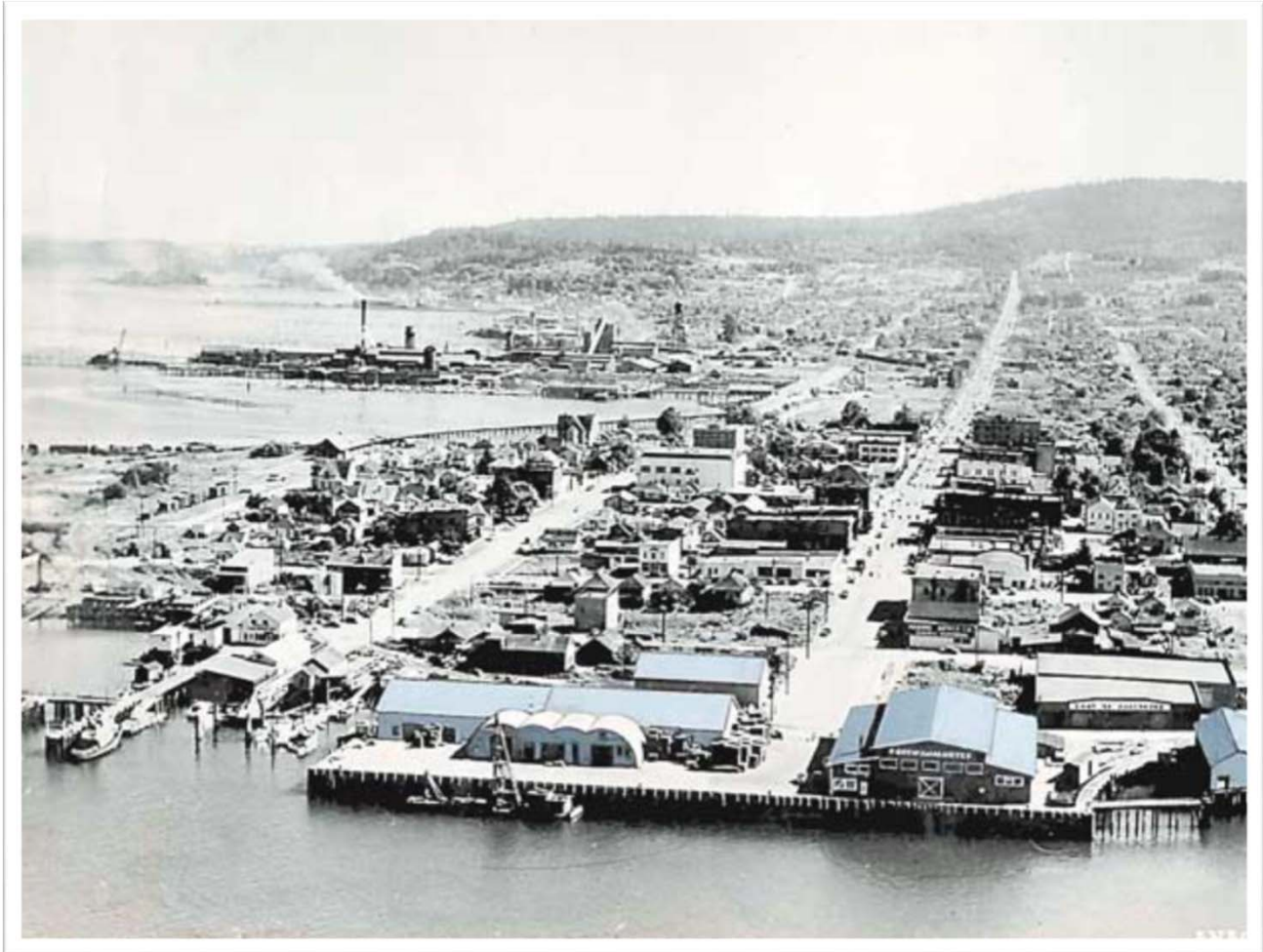
Circa 1946 aerial photograph of Pier 1 and east adjacent Dakota Creek Industries Site along the Guemes Channel shoreline (courtesy of Port of Anacortes).
