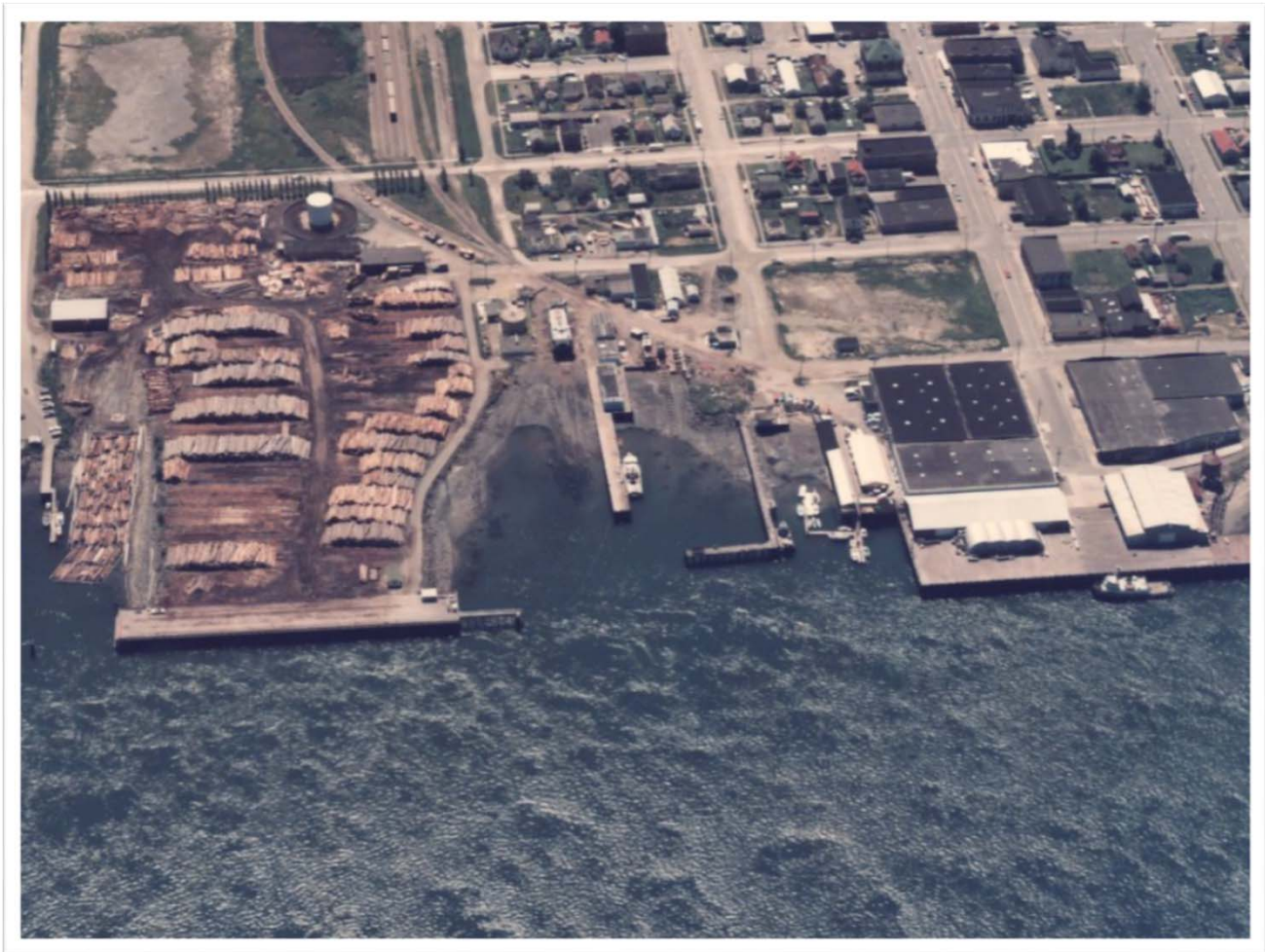
Circa 1977 aerial photograph of the Dakota Creek Industries Site along the Guemes Channel shoreline (Washington State Department of Ecology – Costal Atlas).
