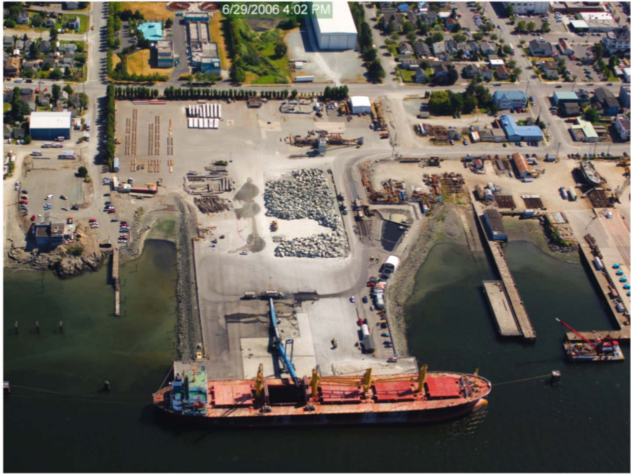
Circa 2006 aerial photograph of the Pier 2 and west adjacent Dakota Creek Industries Site along the Guemes Channel shoreline (Washington State Department of Ecology – Costal Atlas).
