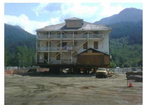
Temporarily moving the Skykomish Hotel, 2009
