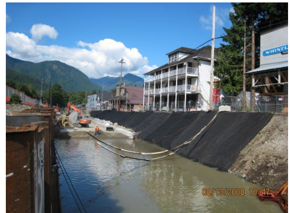
HCC System construction on Railroad Avenue, 2008
