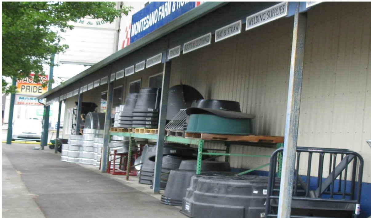
Photo 7: Store building and walkway – from the South.
