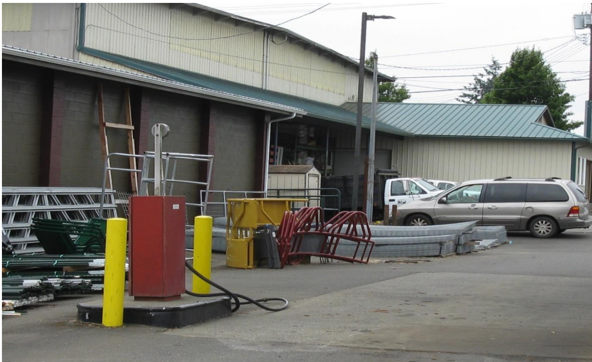
Photo 6: Loading dock and asphalt cap – from the Northeast.
