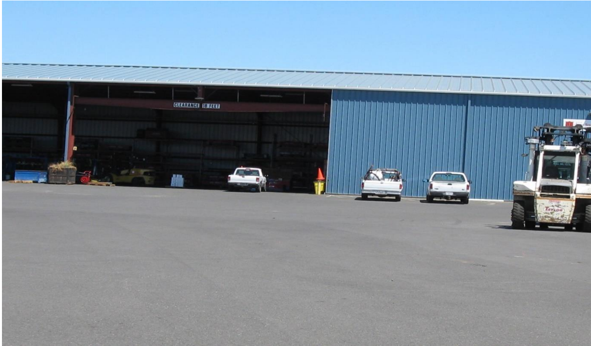
Photo 1. Former pond area and engineered asphalt cap and new building—from the Southeast.
