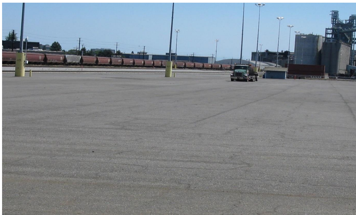
Photo 5: Former plant area and engineered asphalt cap—from the Northwest.
