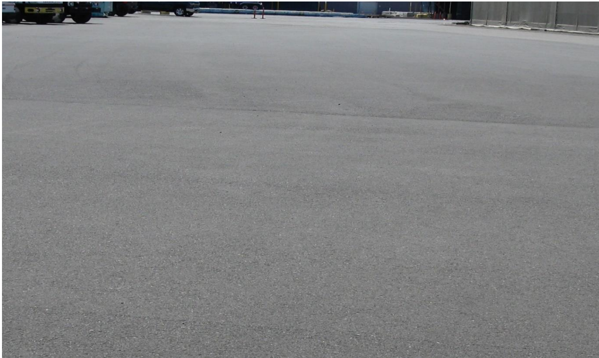
Photo 3. Former pond area and engineered asphalt cap—from the West.
