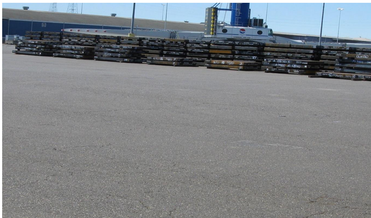
Photo 7. Former plant area and engineered asphalt cap/current storage area—from the Southwest.
