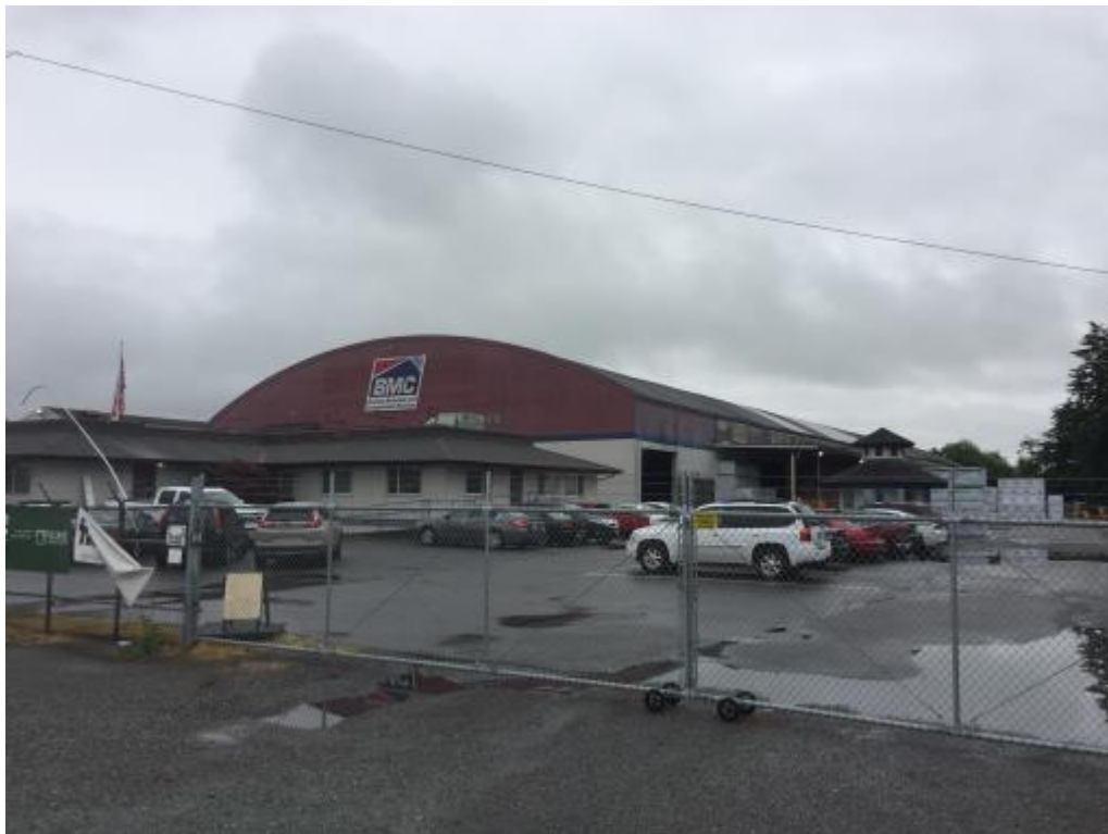
Photo 24 View of the northwest-adjointing Building Materials & Construction Solutions property from 35th Ave NE facing northeast
