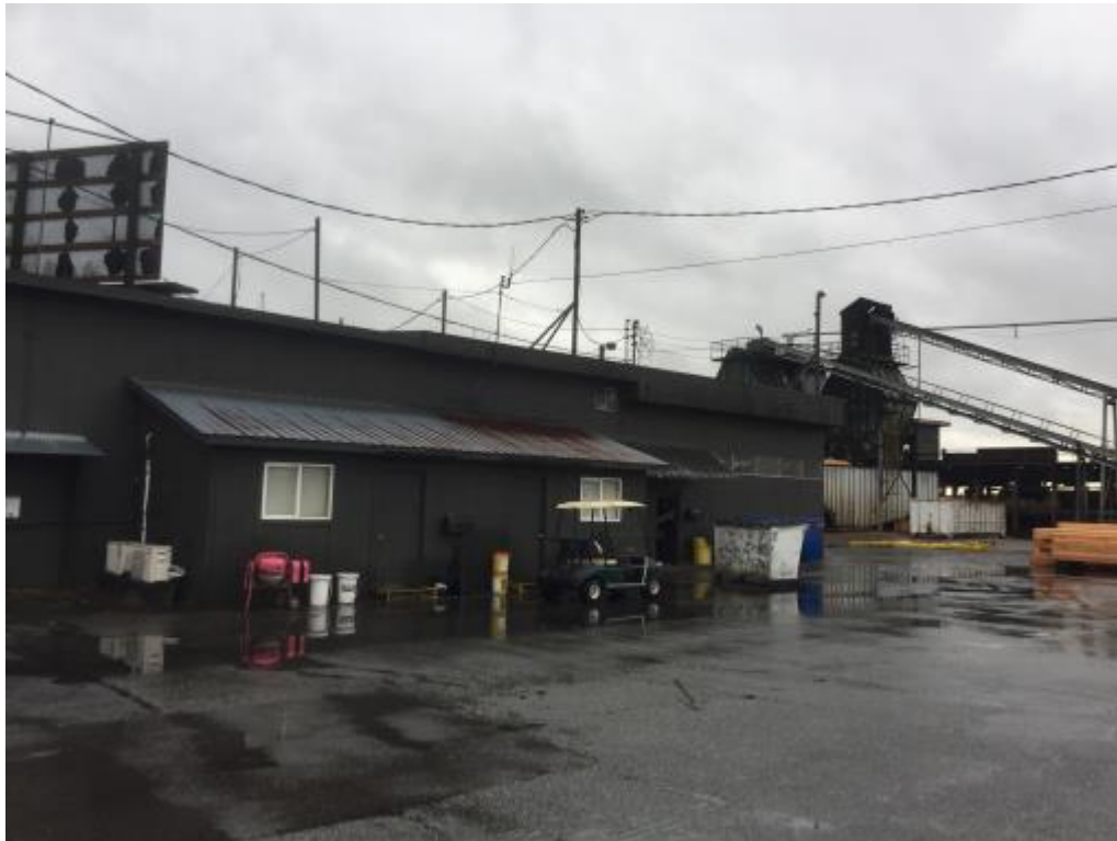
Photo 9 View of the vehicle maintenance building facing southeast
