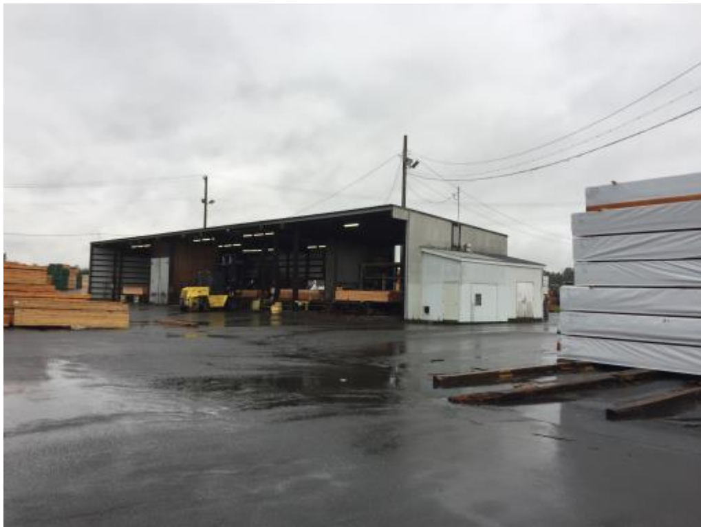
Photo 4 View of the Dip Tank and Bander building facing southwest
