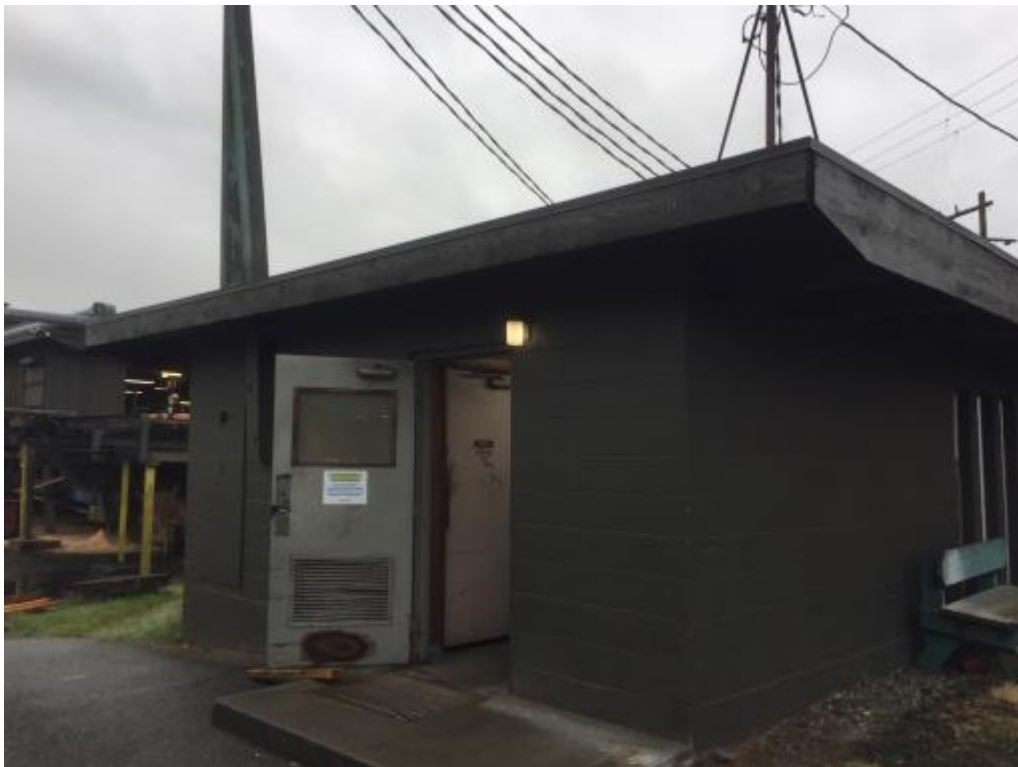
Photo 14 View of the restroom building facing south-southeast
