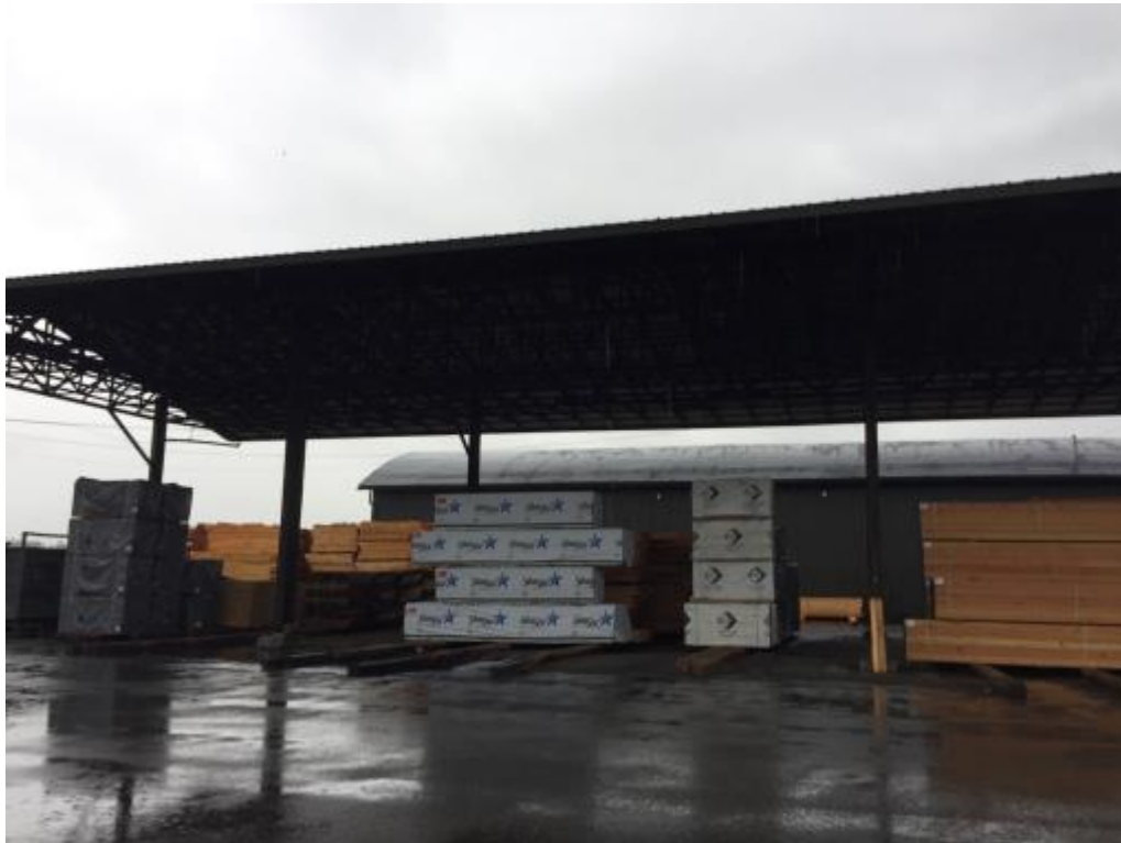
Photo 3 View of the Dry Shed facing east
