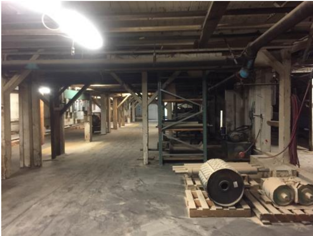
Photo 13 Inside of the saw mill building
