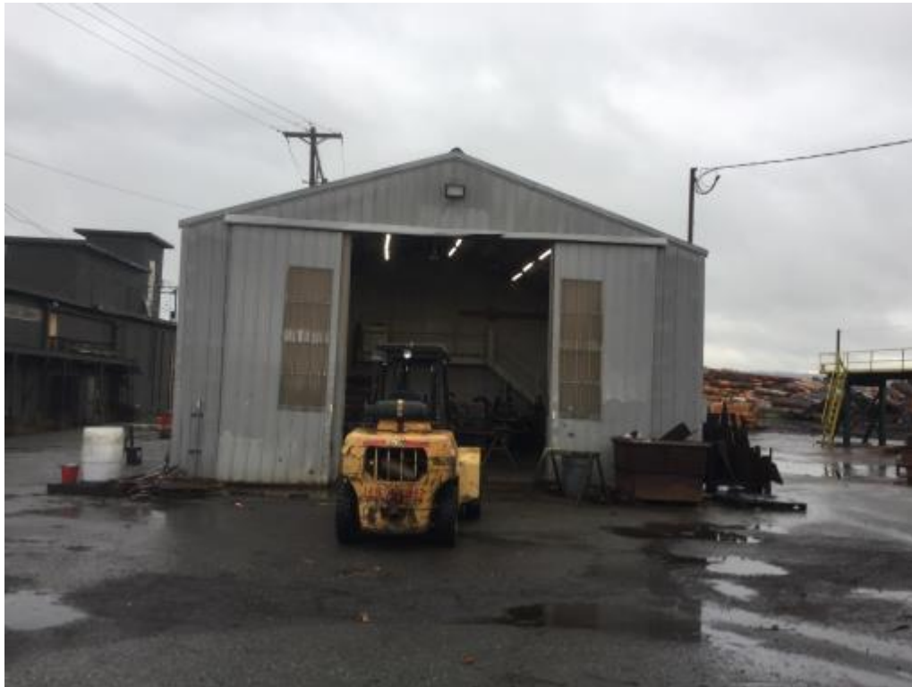
Photo 15 View of the mechanics shop facing east
