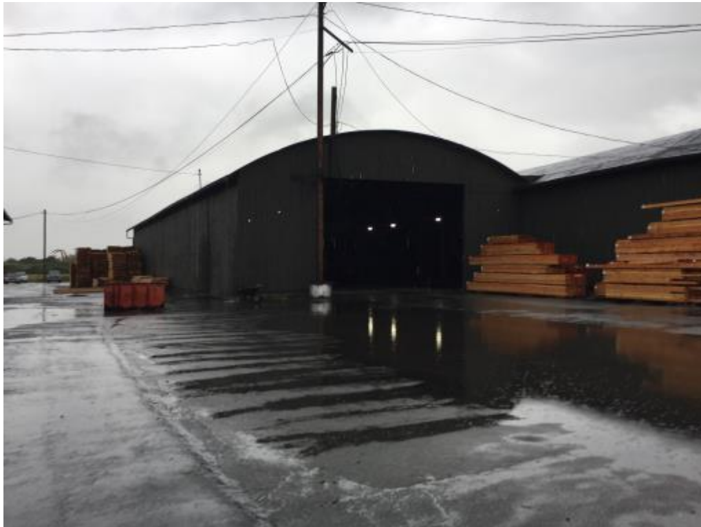
Photo 5 View of the dry storage building facing north-northeast
