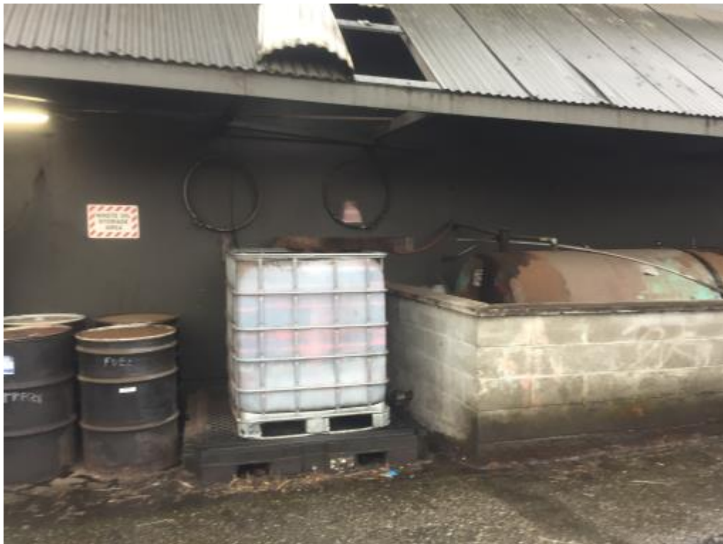
Photo 10 View of the waste oil AST and containers on the north side of the vehicle maintenance building
