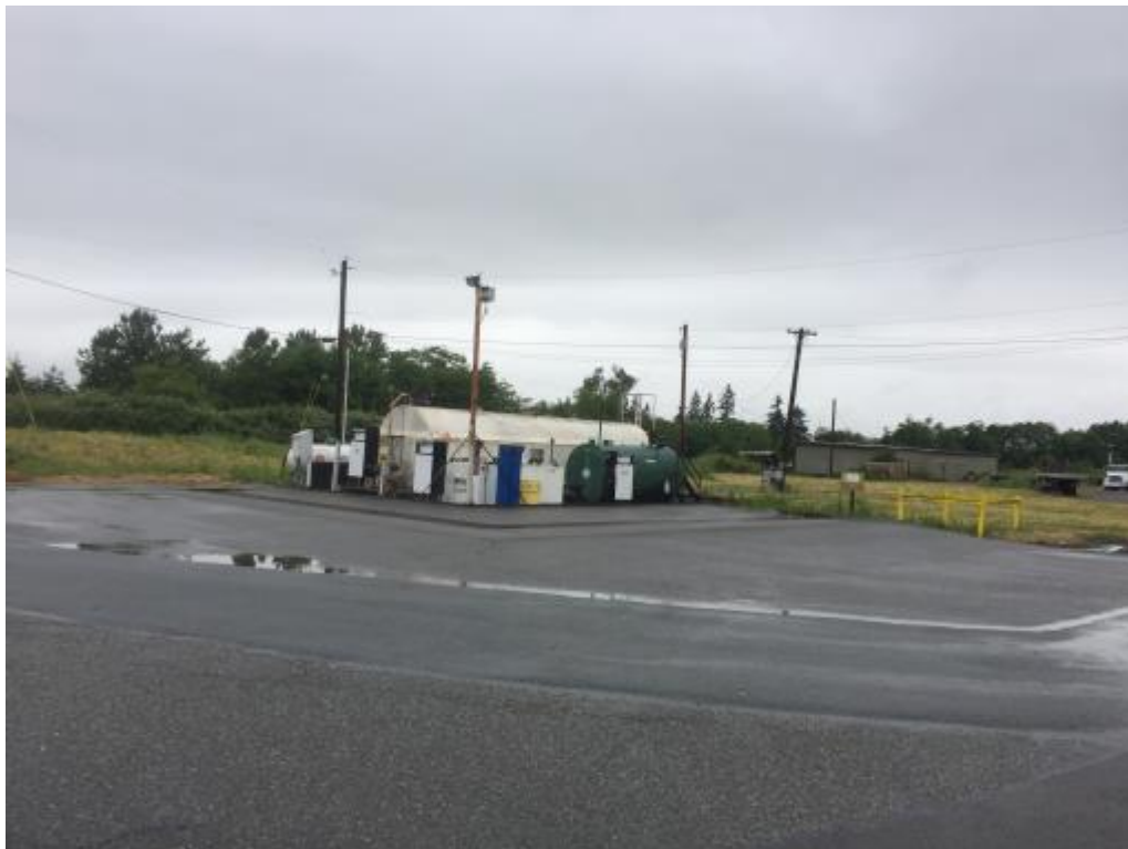
Photo 20 View of the ASTs at the entrance facing northwest
