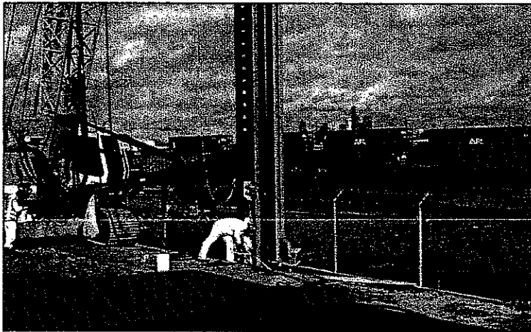
Phase 2 cleanup using bioremediation and extraction pumping to remove petroleum from groundwater and saturated soils in July 2001.
