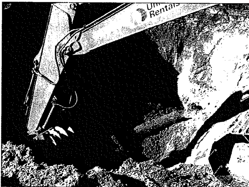
Excavation of soils during phase 1 cleanup in October 2003.
