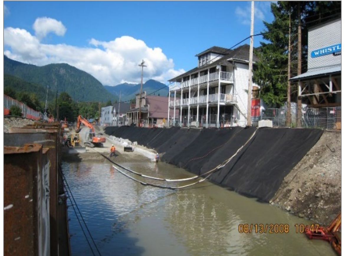
HCC System construction on Railroad Avenue, 2008
