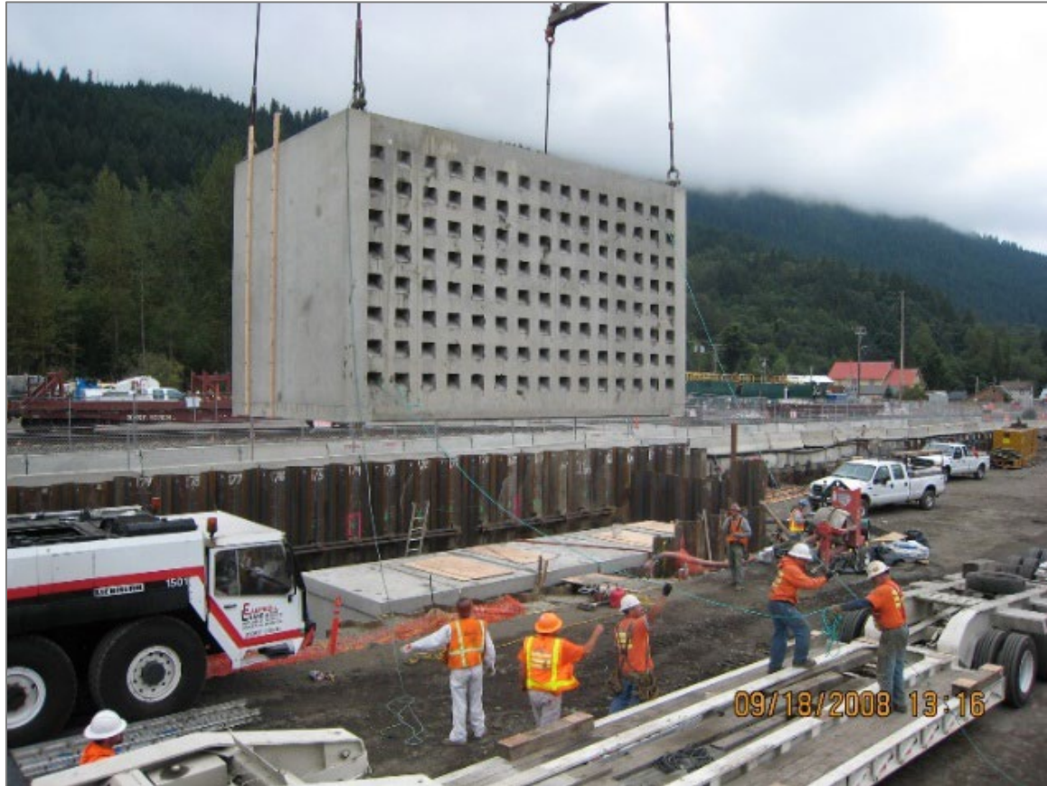
Installation of HCC treatment gate system, 2008
