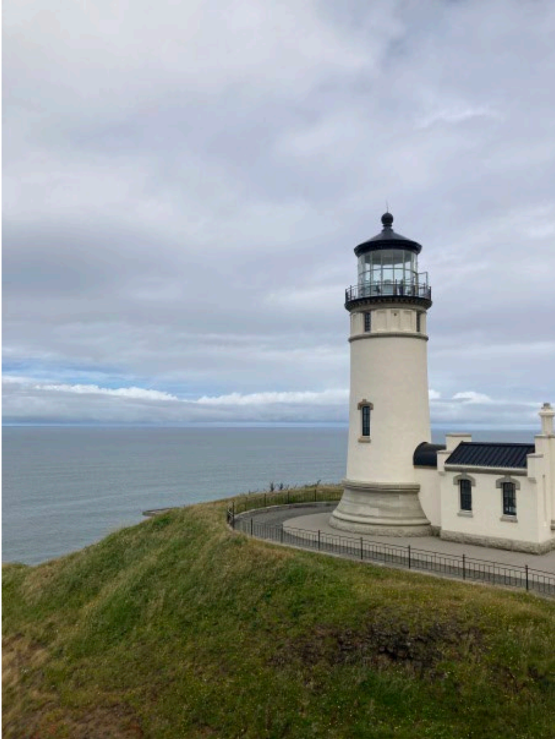
Photo 1: View of the Lighthouse from the Southeast (view to the northwest)
