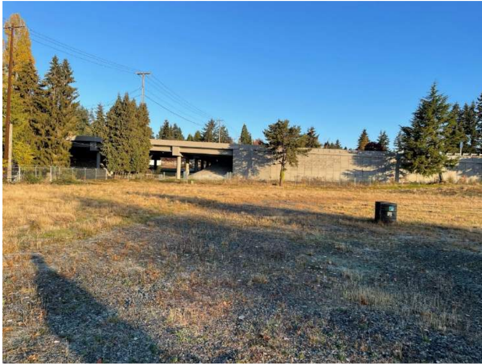
Photograph 1. Area near the northwest corner of the property after landscaping and cutback of noted plant overgrowth.
