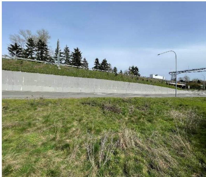
L10. Fair conditions with some plant overgrowth at Station WSDOT-10.
