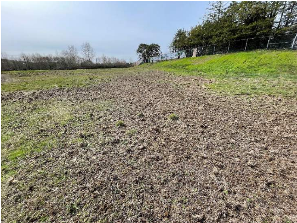
Photograph L6. Large area at the southwest portion of the property near Stations LLA 12 and LLA 18 with noted loss of vegetation used for erosion control.
