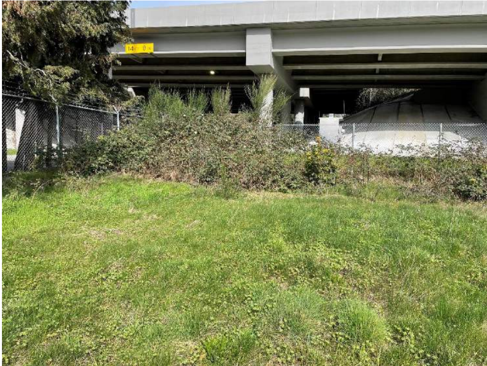
Photograph L3. Station LLA 07 and LLA 08, at the northwest corner of the property, with notable plant overgrowth.
