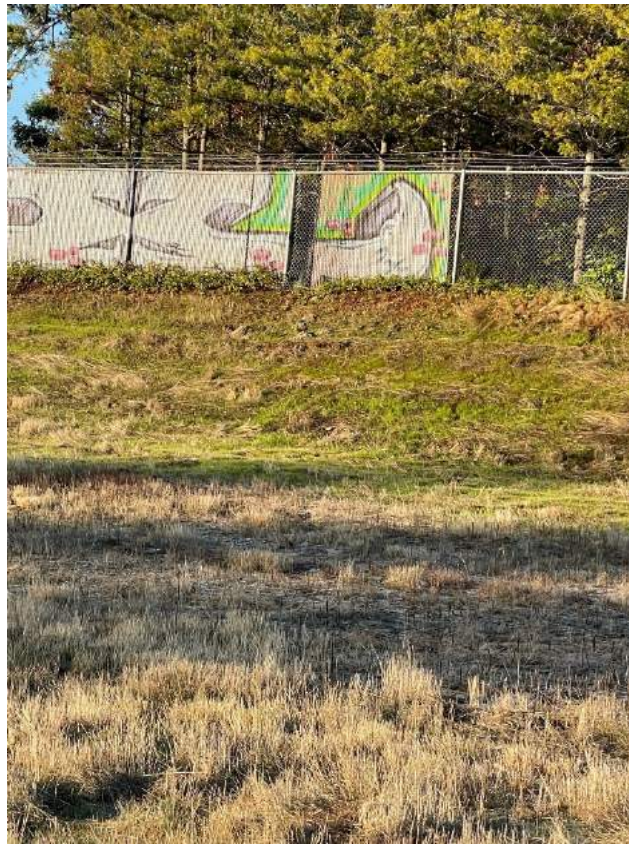
Photograph 3. Fence repairs along the southern portion of the west fence line.
