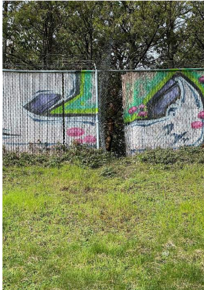
Photograph L7. Removed fence panel near Station LLA 12.
