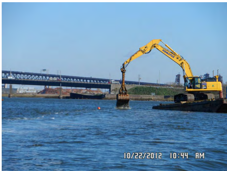
Photo 1: Mechanical placement of armor in Cap Area 17.
