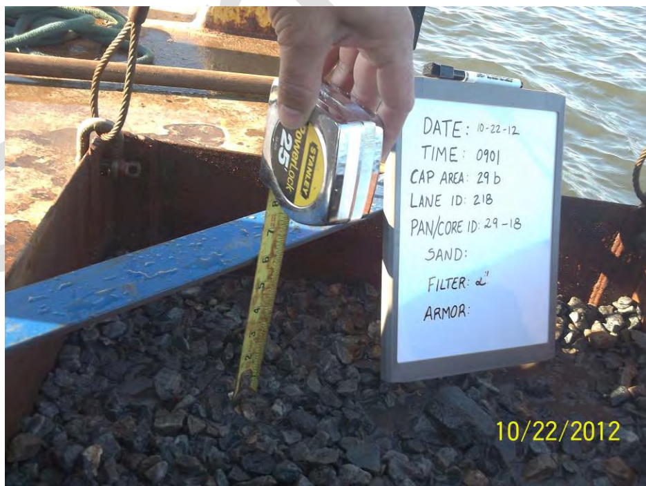
Photo 2: Filter thickness verification in Cap Area 29B.
