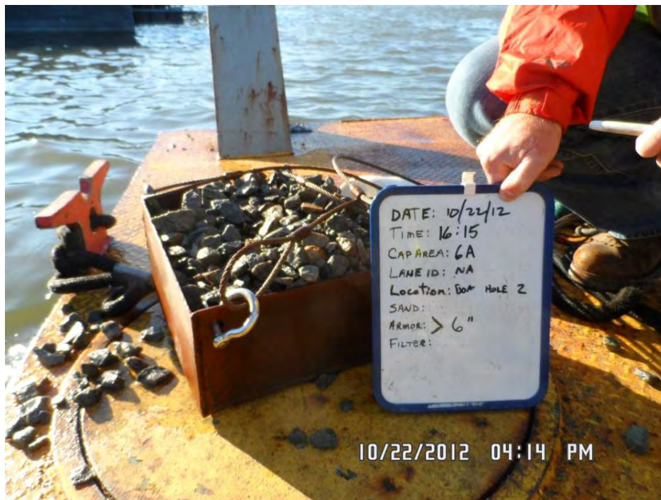
Photo 3: Armor thickness verification in Cap Area 6A.
