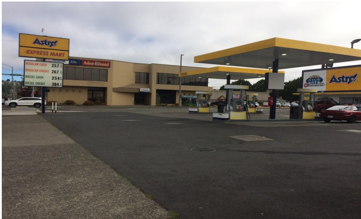
Photo 3: Pump Islands and Asphalt Cap From the Northwest.
