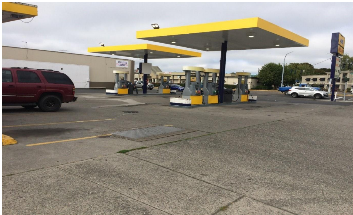
Photo 4: Pump Islands From the Southeast.
