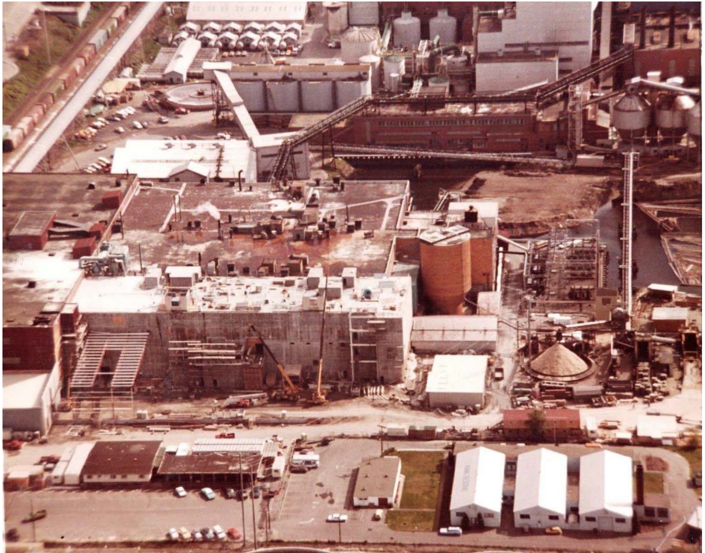
Photograph 1. Initial filling of Log Pond, viewed from the north (ca. 1979). The initial wedge of fill visible is also where geophysical anomaly (D) is located (refer to Attachment A text).
