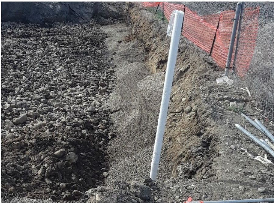
Photograph 46. Installation of westernmost bioventing line on Toad's property. View S.
