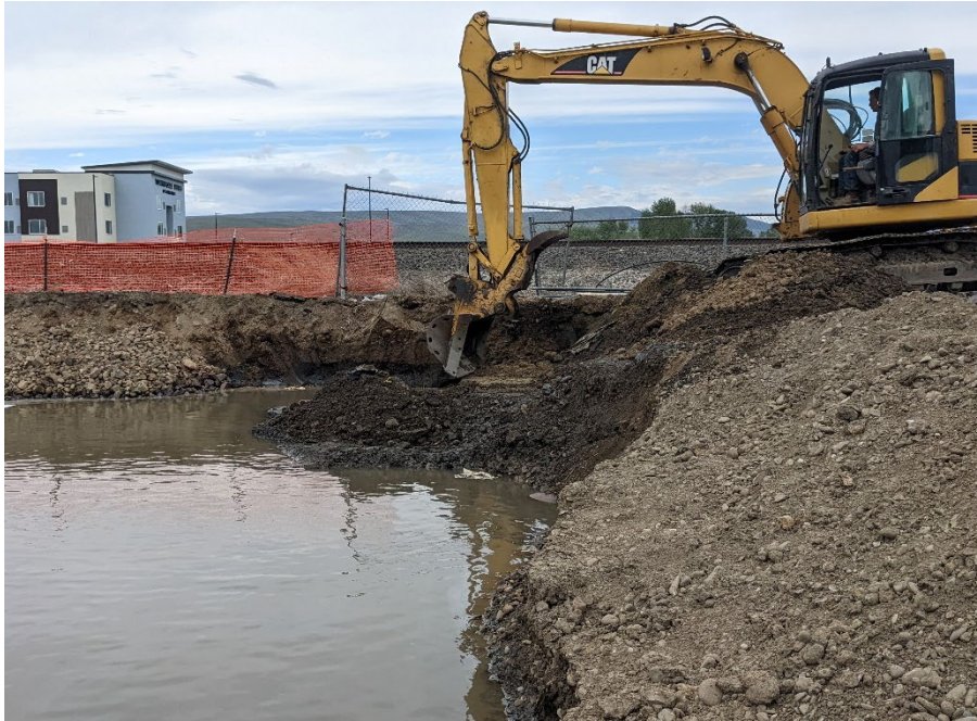
Photograph 35. Overexcavation of LNAPL collection trench. View W.
