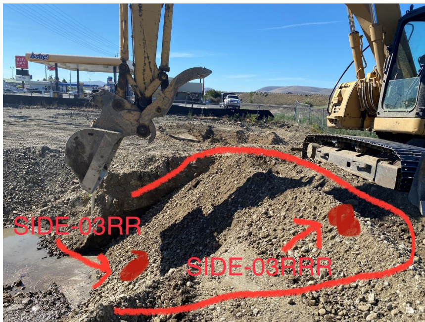
Photograph 8. Sampling locations of SIDE-03RR and SIDE-03RRR after being backfilled. View SW.
