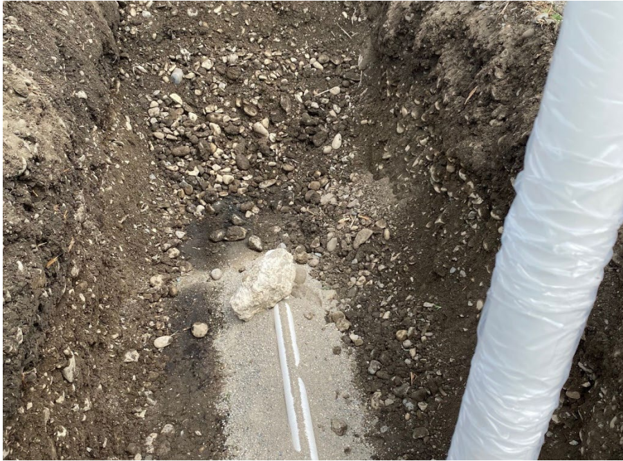
Photograph 49. Installation of horizontal bioventing injection point.
