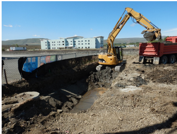
Photograph 2. Excavation along Toad's property boundary. View SW.
