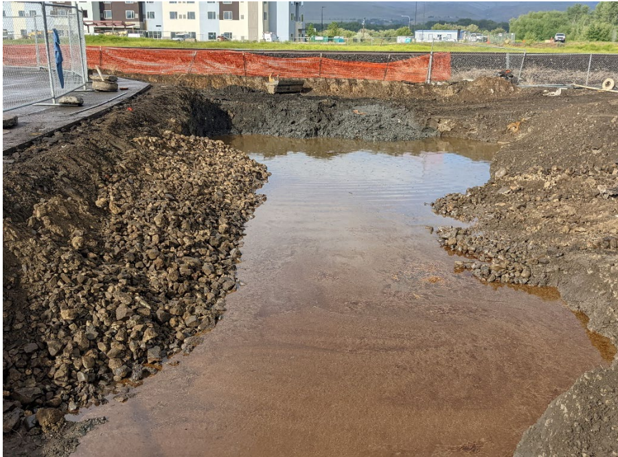
Photograph 31. Post-excitation slope shoring along Toad's property. LNAPL in excavation emerged during removal of LNAPL collection trench pea gravel that was still present on the southern end of the Big B property. View W.
