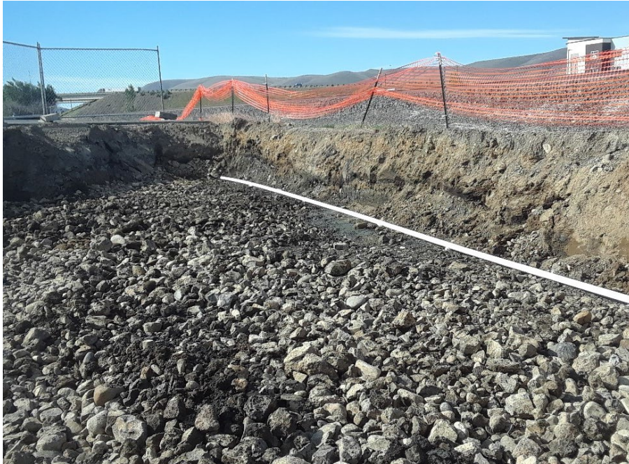
Photograph 45. Installation of westernmost bioventing line on Toad's property. View SW.
