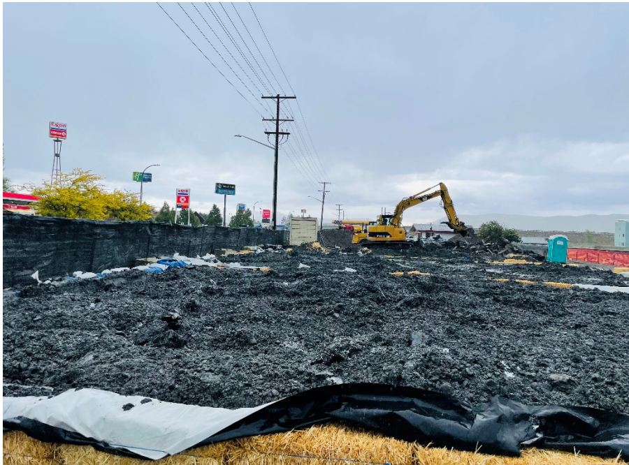
Photograph 15. Mixing of impacted soil to prepare for landfarming. View S.
