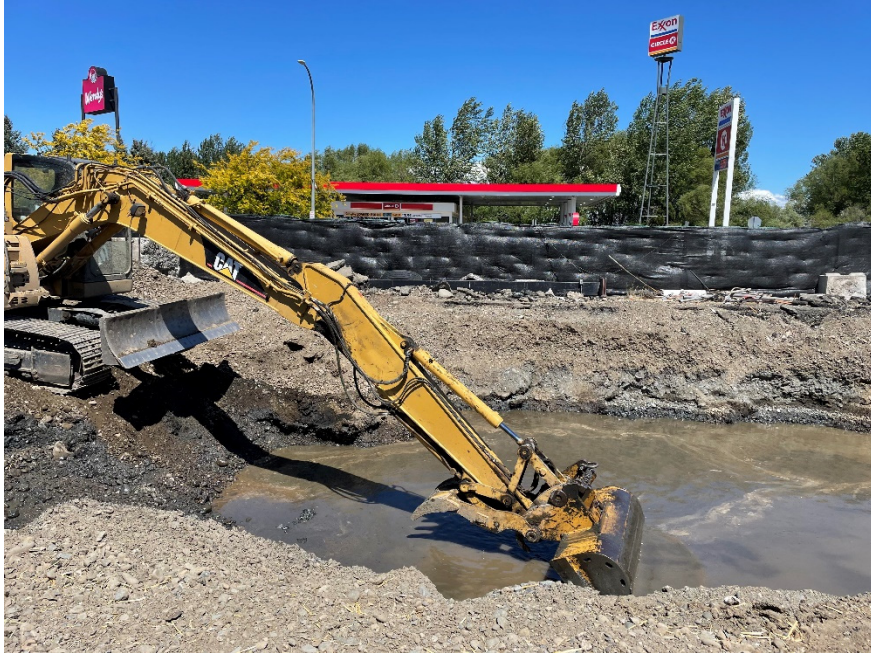
Photograph 9. Gasoline-range organics (GRO) excavation. View E.
