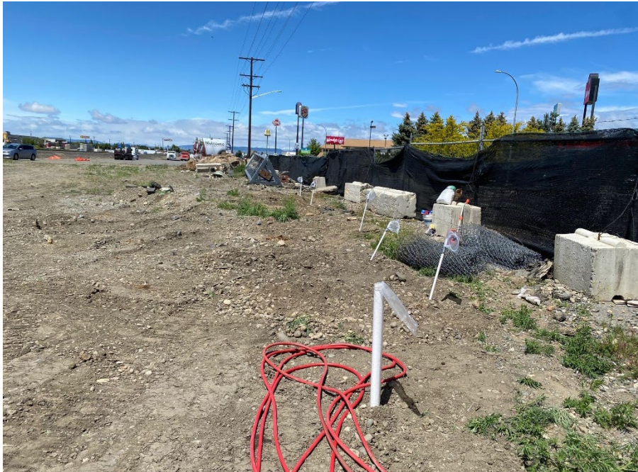
Photograph 57. Final locations of injection point (foreground) and soil vapor monitoring points. View N.
