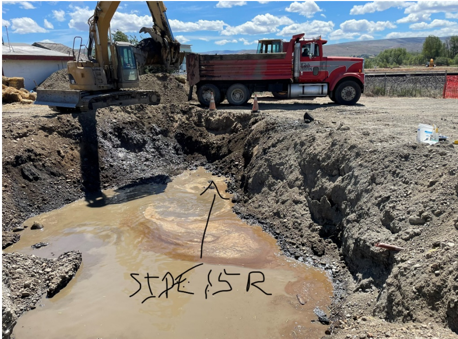
Photograph 13. Sampling location of SIDE-15R within northern DRO excavation. View SW.
