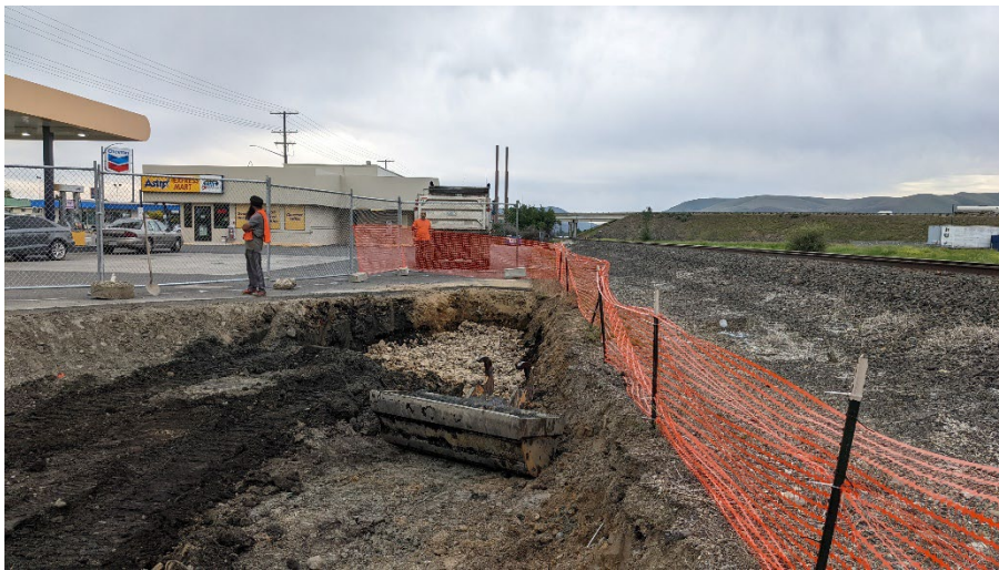
Photograph 32. Excavation and slope shoring in BNSF ROW. View S.
