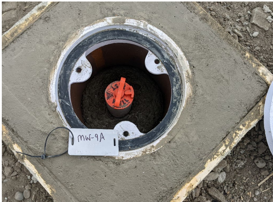
Photograph 52. Monument completion of MW-9A.
