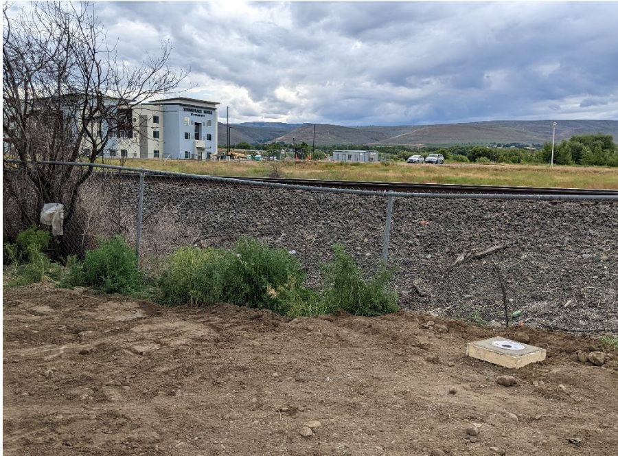
Photograph 53. Monument replacement of MW-3. View SW.
