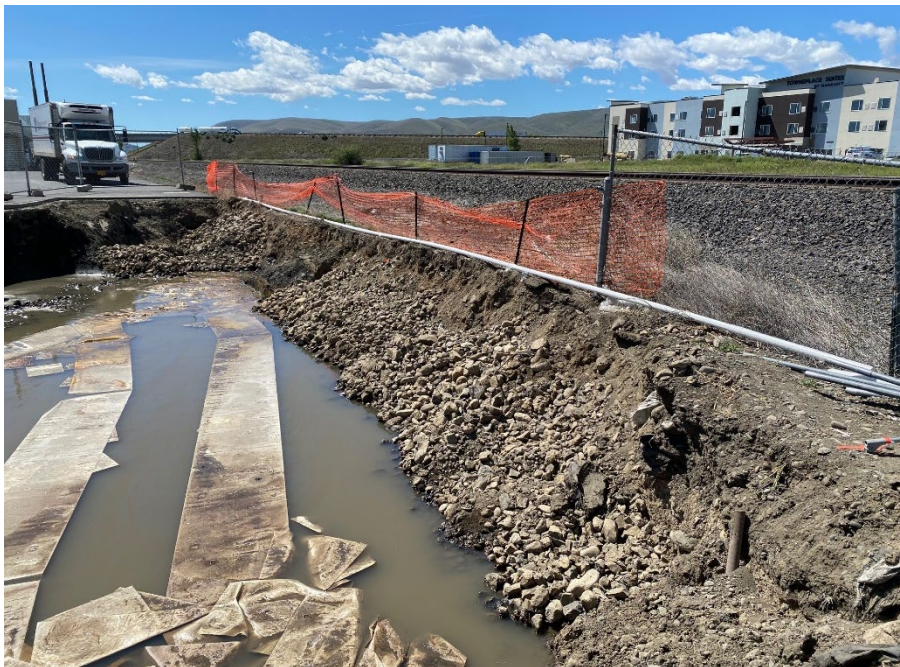
Photograph 36. Slope stabilization and adsorbent material in BNSF ROW. View S.
