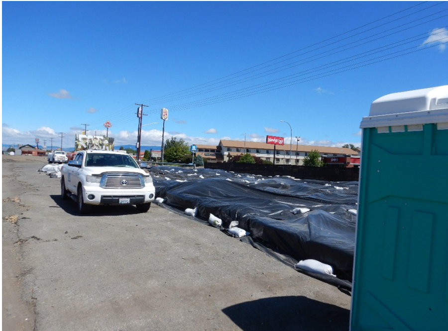
Photograph 17. Covered landfarming area. View NE.
