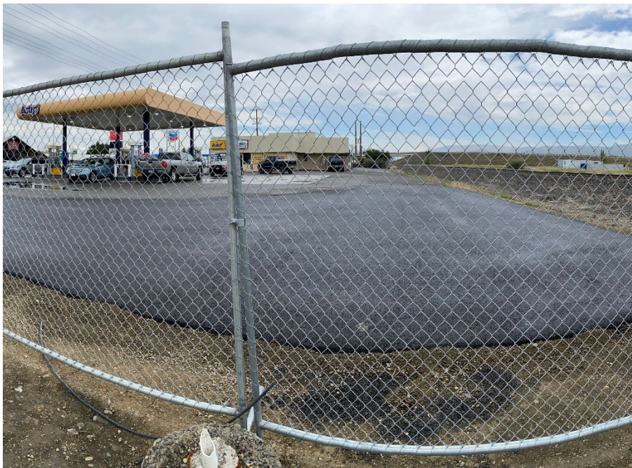
Photograph 48. Final paved surface on Toad’s property. View S.
