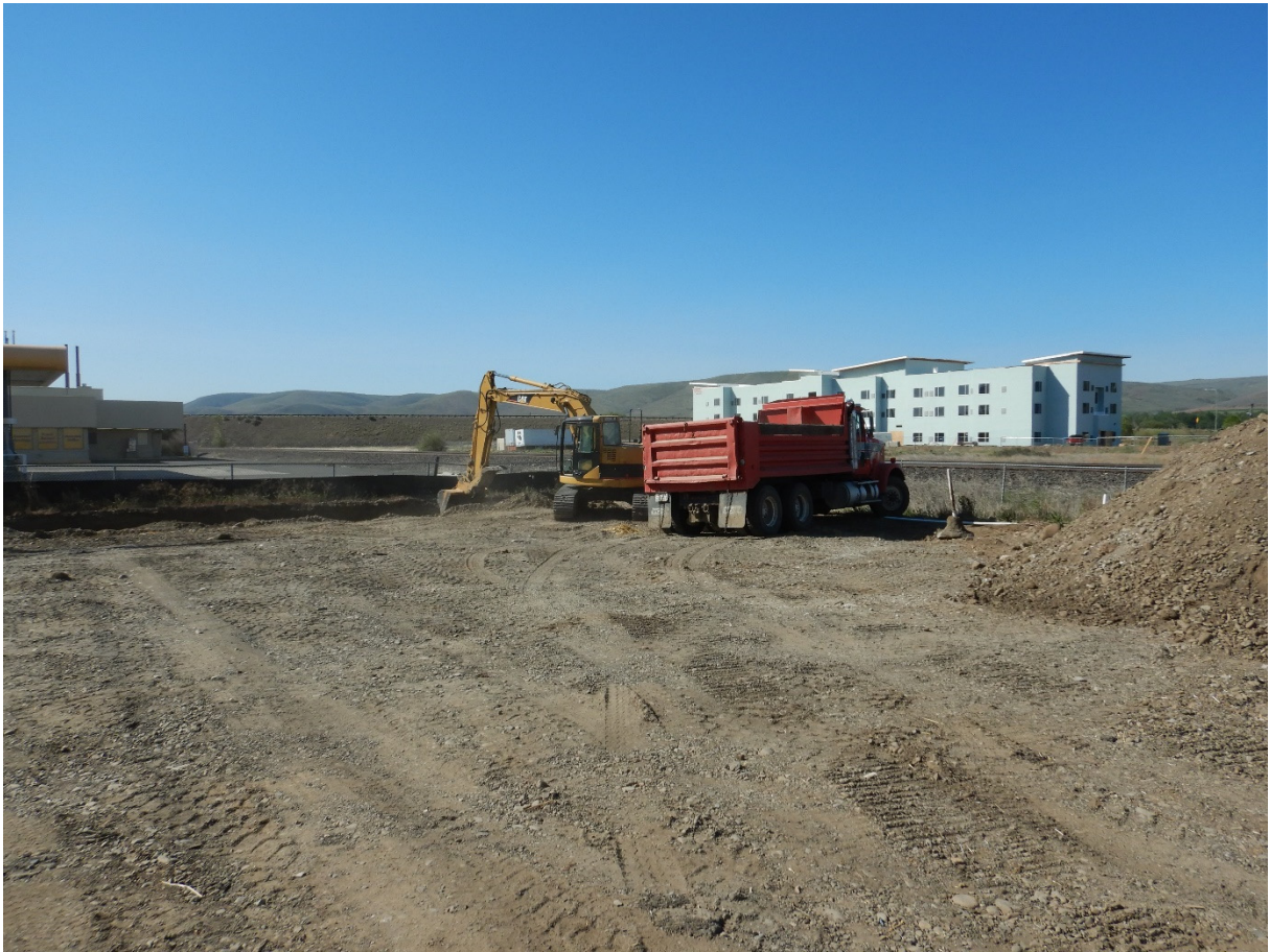
Photograph 1. Overburden removal in southern diesel-range organics (DRO) excavation area. View SW.
