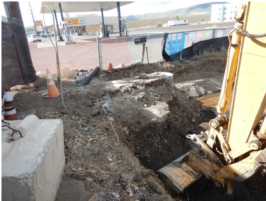
Photograph 4. Excavation above sewer line. View S.
