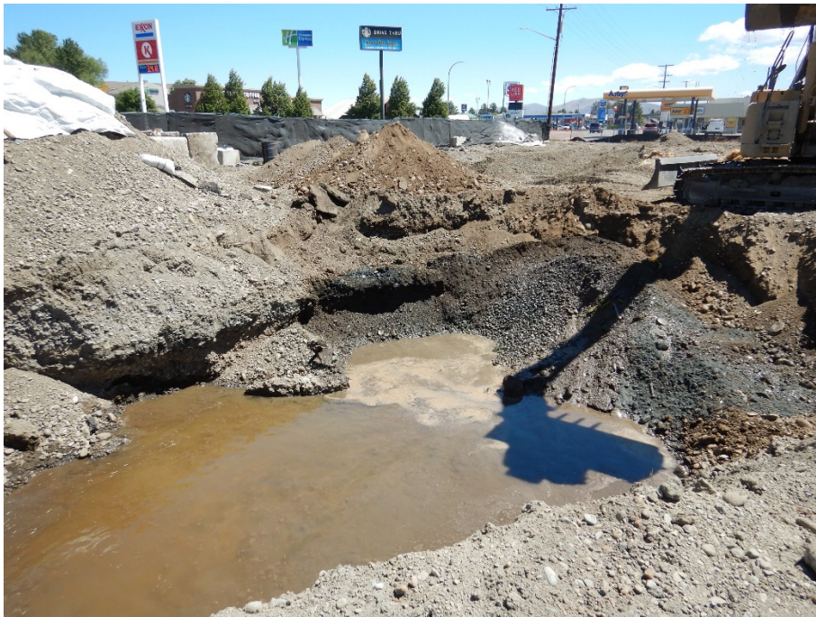
Photograph 12. Northern DRO excavation. View SE.
