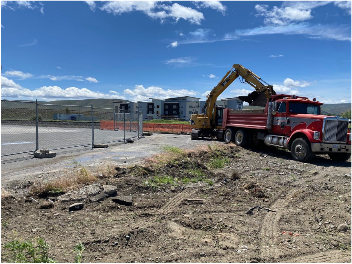
Photograph 21. Toad's property asphalt removal and fencing extent. View SW.
