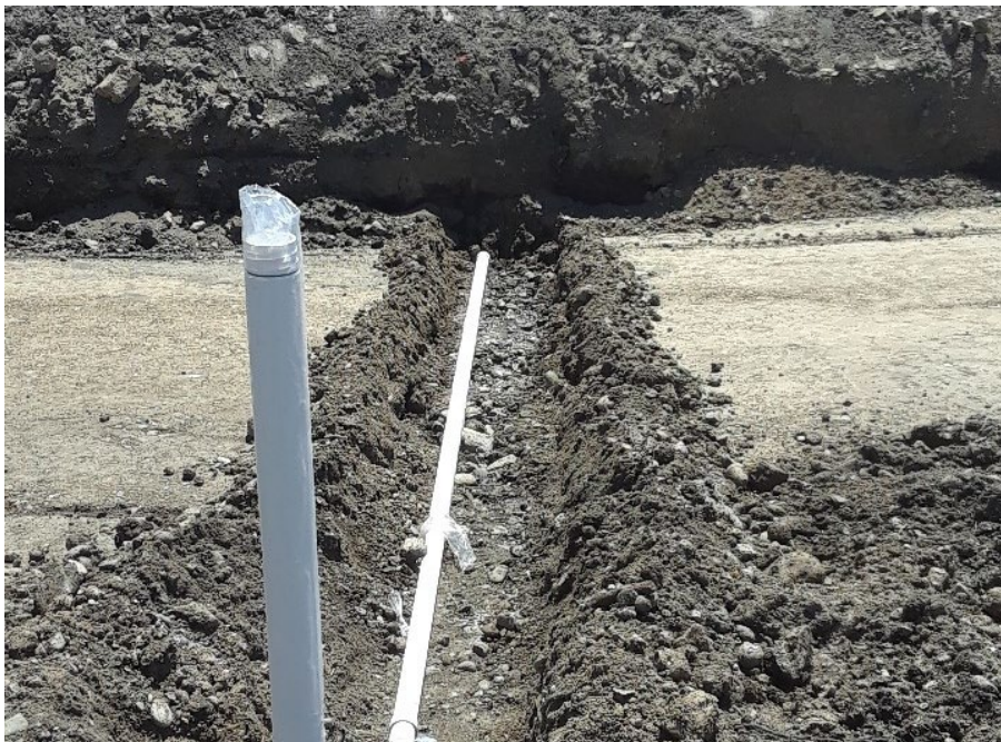
Photograph 44. Installation of center Toad's property bioventing line. View S.
