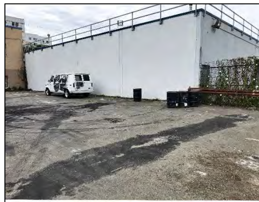
Photo 6: Post operation site.
