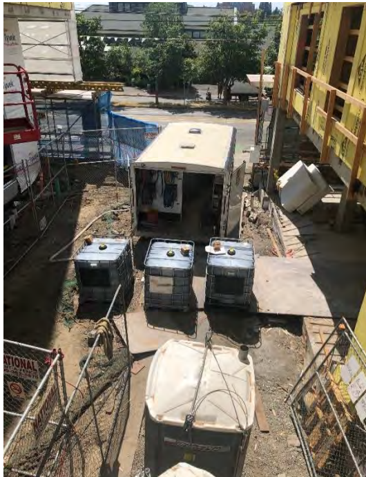
Photo 3: RRS Injection Trailer and staged PlumeStop totes (South View)
