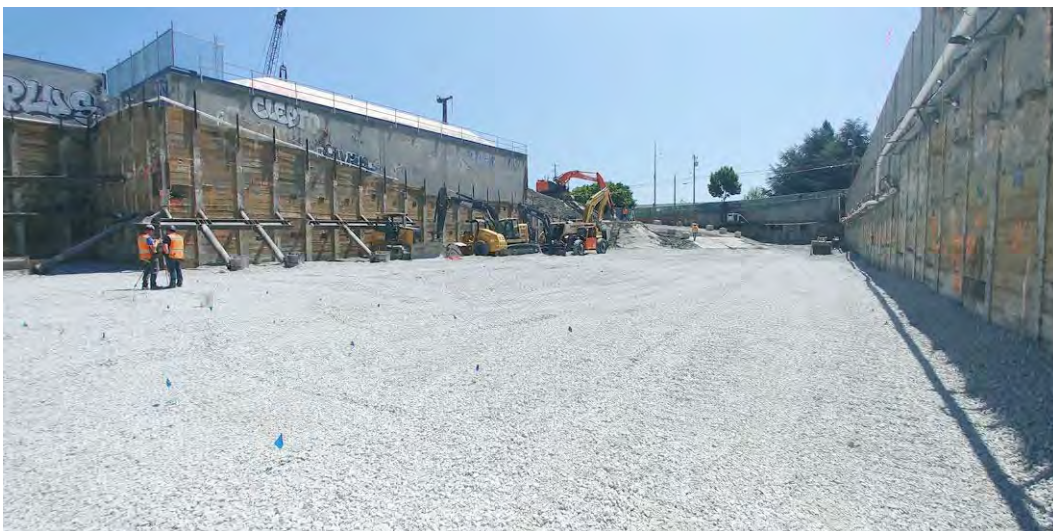
44. View of the main excavation with a gravel base layer installed.
