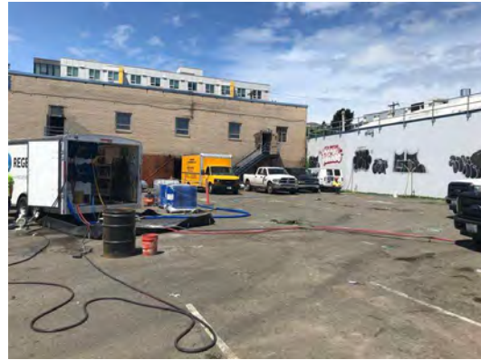
Photo 2: Injection trailer location.
