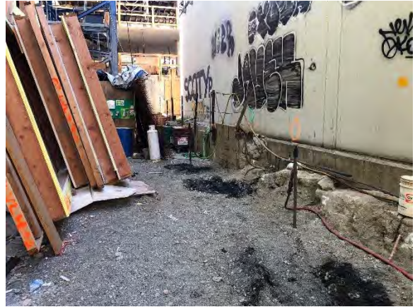
Photo 2: Injection Area. (West View)
