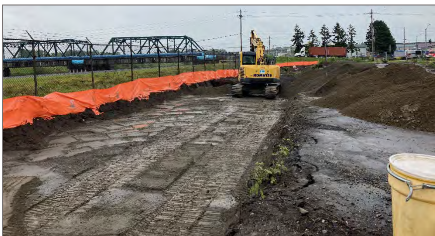
Photo 1: Wet backfill as observed today in UP-22. Photo faces southeast.
