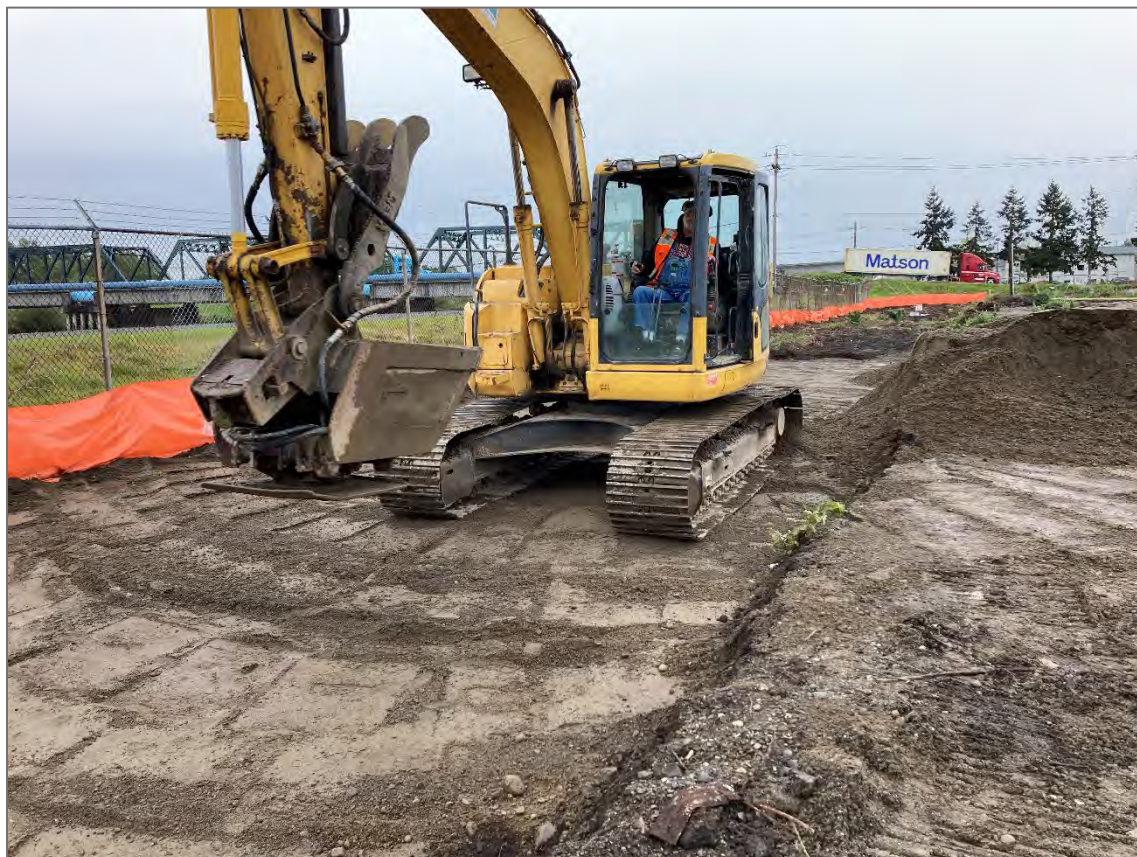
Photo 1: Backfill as observed today in UP-22. Photo faces southeast.
