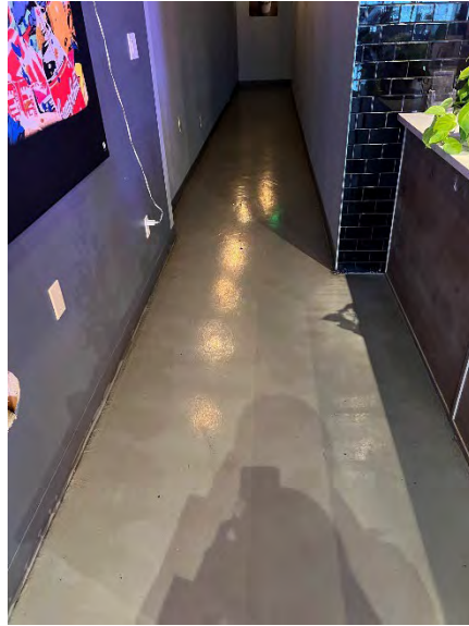
Photograph 11. Floor Slab in Adjacent-West Tenant Space (Suite B7) (December 19, 2022)
