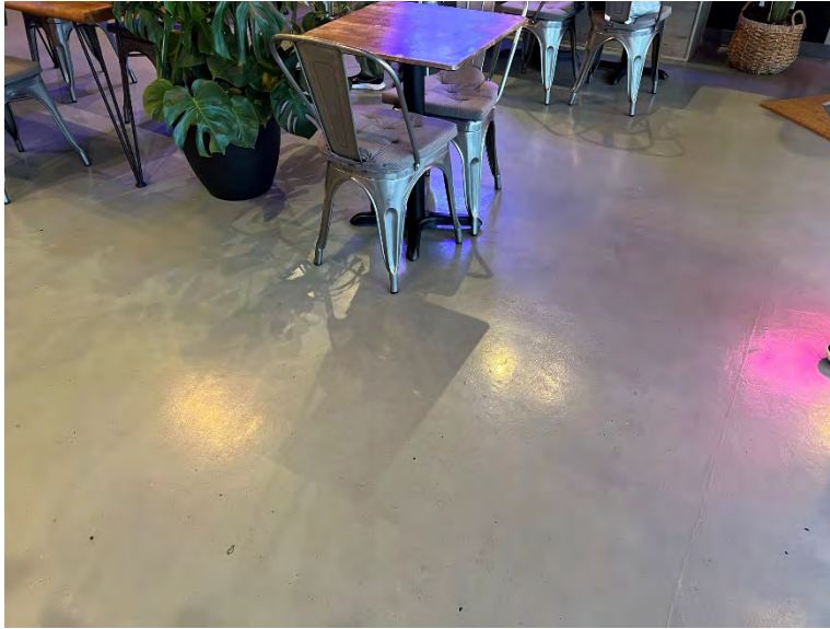
Photograph 9. Floor Slab in Adjacent-West Tenant Space (Suite B7) (December 19, 2022)
