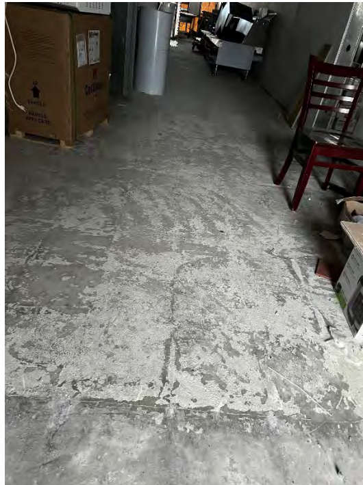
Photograph 19. Floor Slab in Suite B5 (December 19, 2022)
