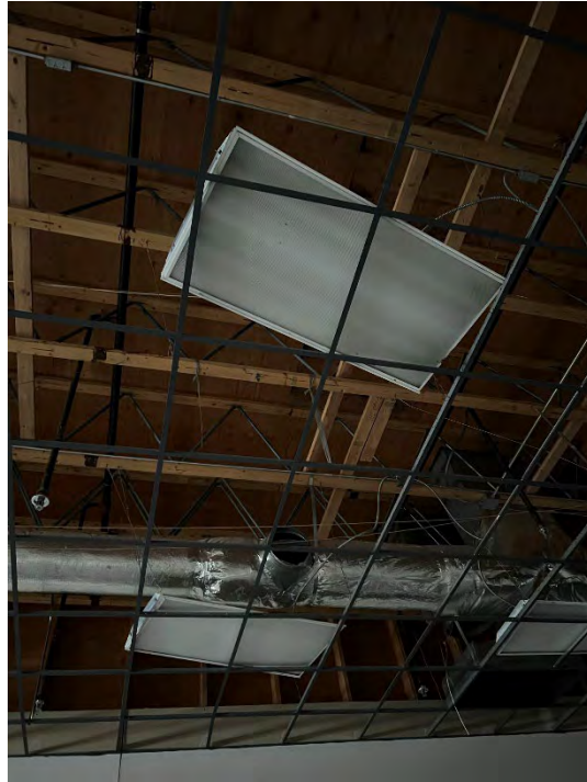
Photograph 7. Dismantled HVAC system of Former Harbour Pointe Cleaners (Suite B6) (December 19, 2022)
