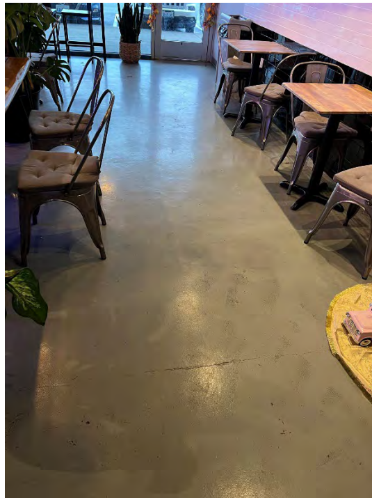
Photograph 8. Floor Slab in Adjacent-West Tenant Space (Suite B7) (December 19, 2022)
