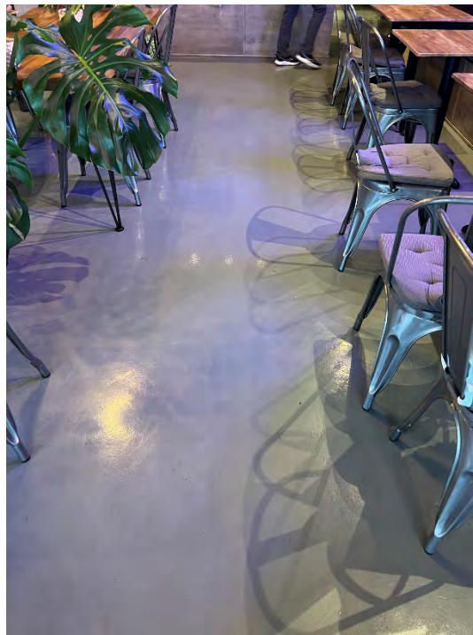
Photograph 10. Floor Slab in Adjacent-West Tenant Space (Suite B7) (December 19, 2022)
