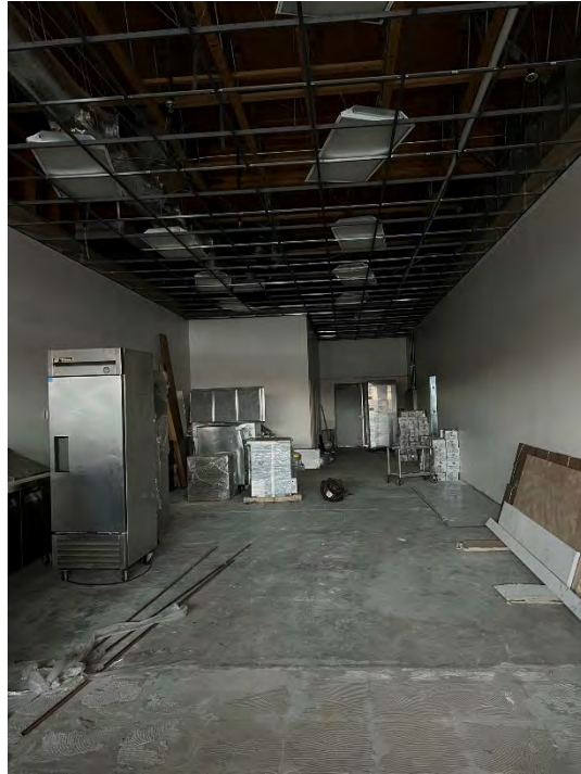
Photograph 1. Floor Slab in Former Harbour Pointe Cleaners (Suite B6) (December 19, 2022)
