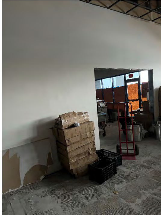
Photograph 5. Floor Slab in Front of Former Harbour Pointe Cleaners, Looking Toward Suite B7 (Suite B6) (December 19, 2022)
