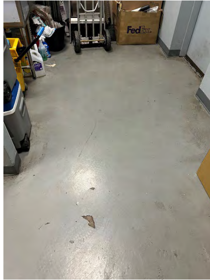
Photograph 13. Floor Slab in Hallway of Adjacent-West Tenant Space (Suite B7) (December 19, 2022)
