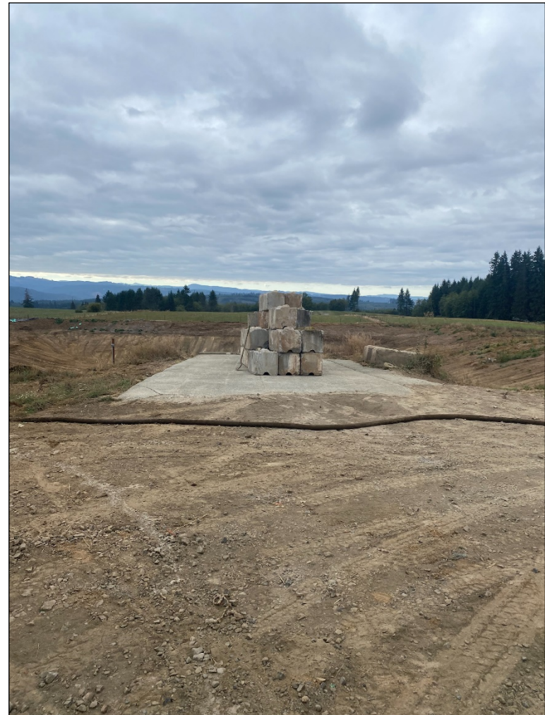
18. 2022: Dump slab loading area (cleaned), looking south.
