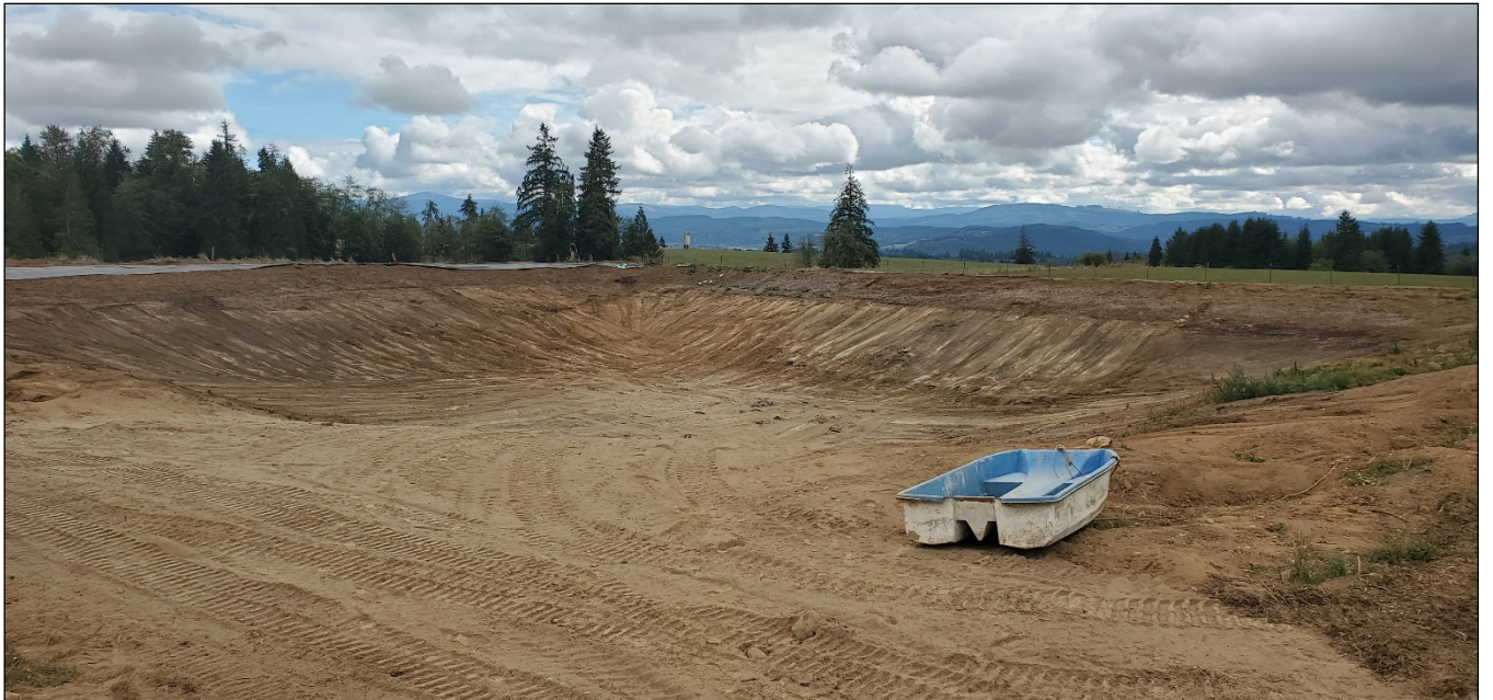
12. 2022: Mixed material removed, looking southeast.
