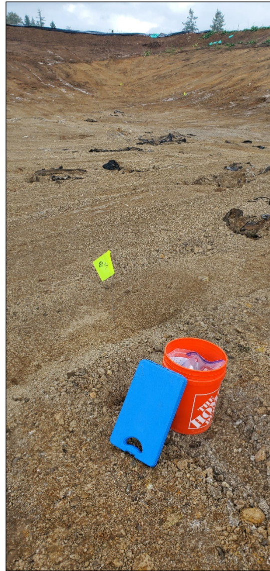
14. 2022: Confirmation sample B4, looking northwest.
