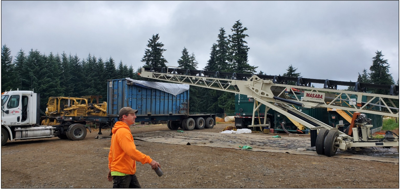
11. 2022: Mixed material conveyed into LeMay containers.
