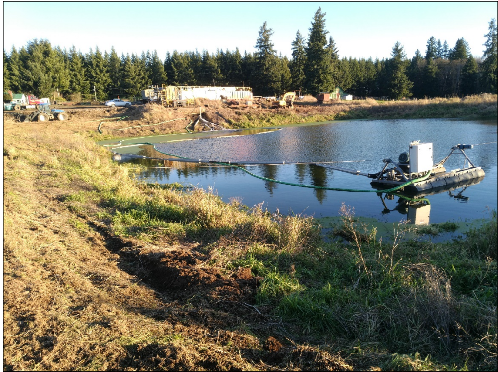
1. 2020: FMF dredge in foreground, centrifuge in background, looking north.
