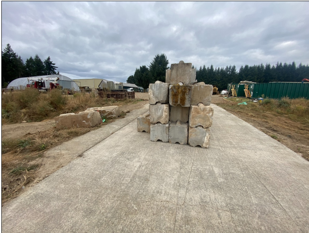
19. 2022: Dump slab truck loading area (cleaned), looking north.
