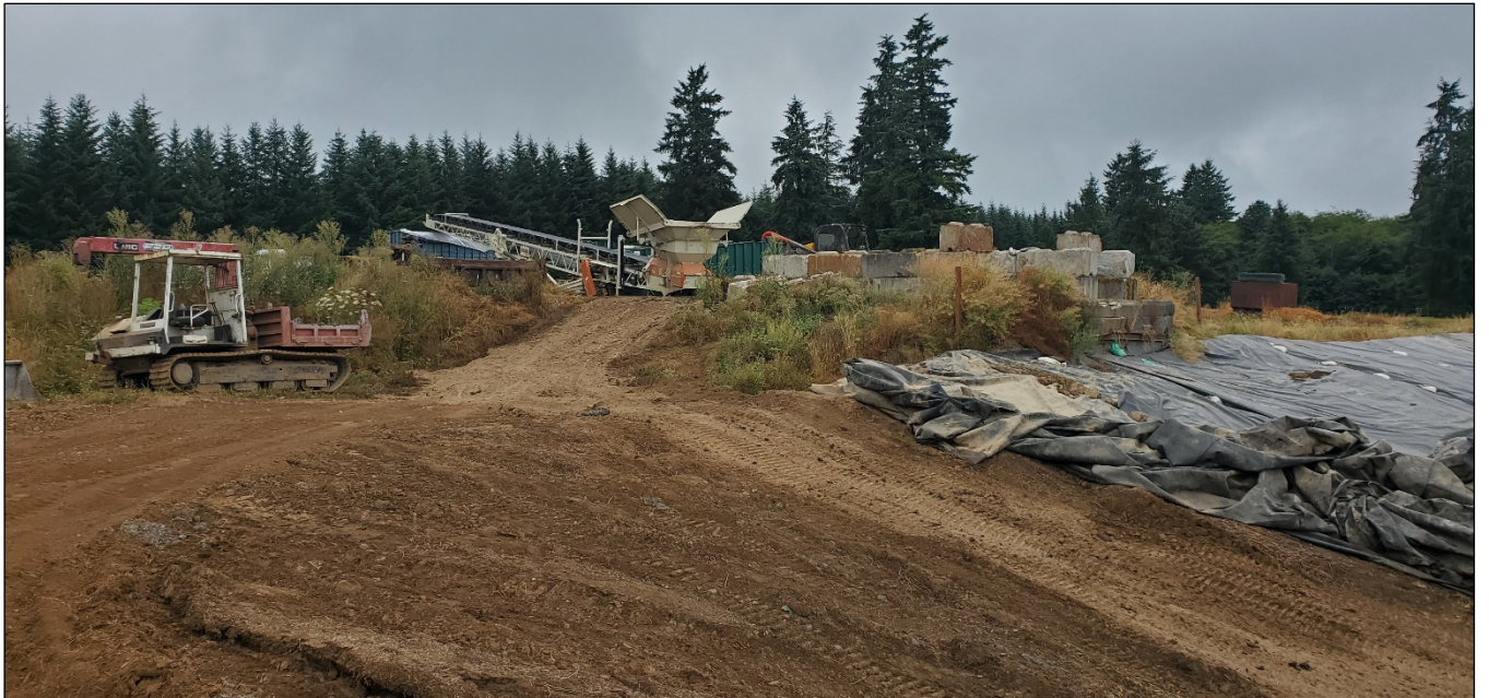
8. 2022: Haul road to conveyor, looking east.
