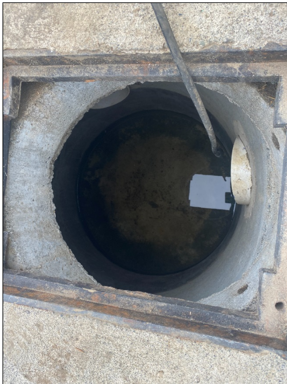
20. 2022: Upland solids staging area, FMF north catch basin after cleaning.
