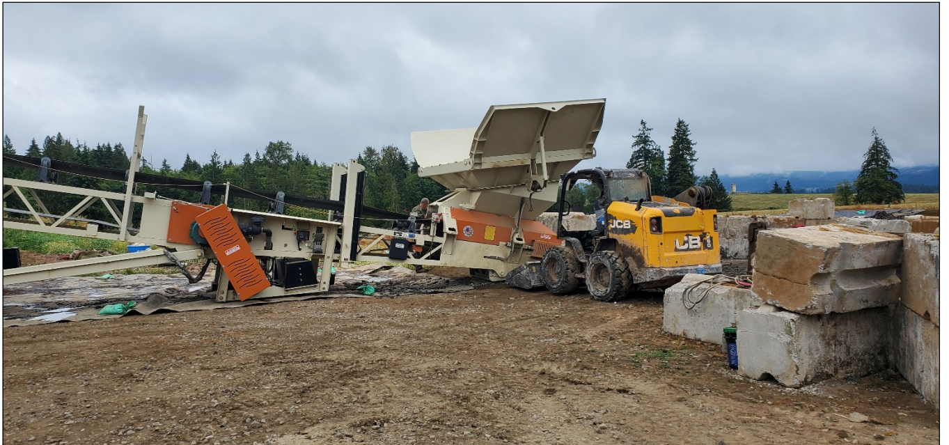
10. 2022: Mixed material being loaded on conveyor.
