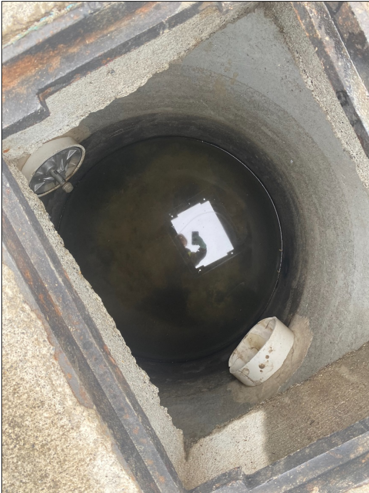
23. 2022: Upland solids staging area, FMF south catch basin after cleaning.
