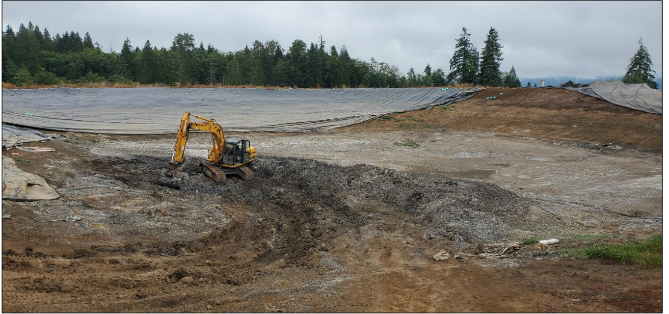
7. 2022: Mixed-material dig excavation, looking southwest.
