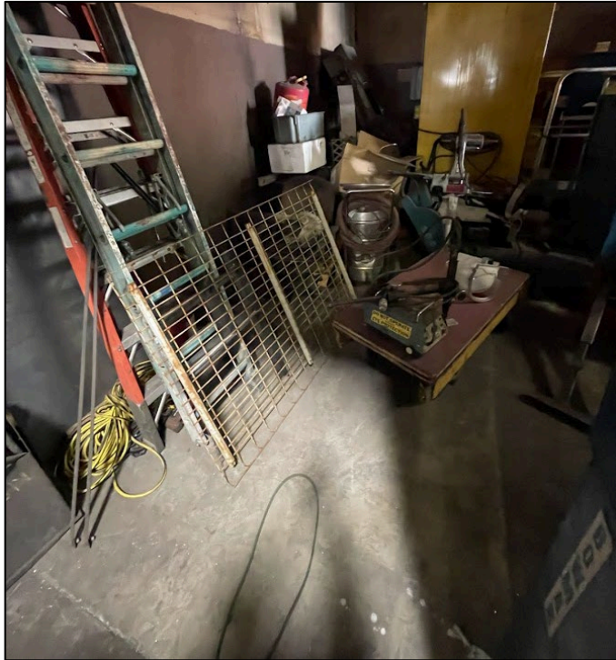
Evaporator pit sealed in April 2020 with heavy equipment stored on top
