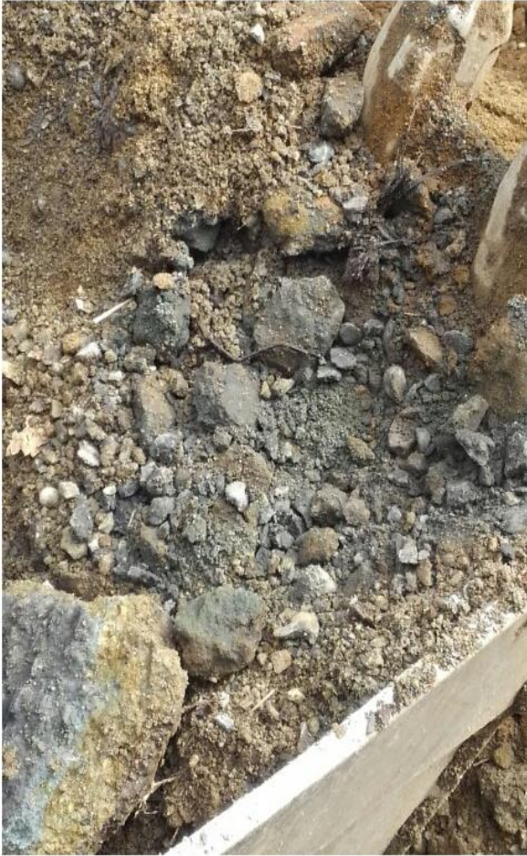
Cleanup of SS-3 Area and confirmation sample area
