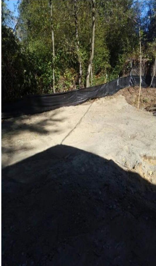
Backfill of front area
