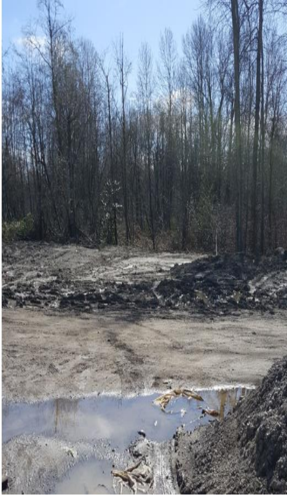
Grading and soil displacement on property
