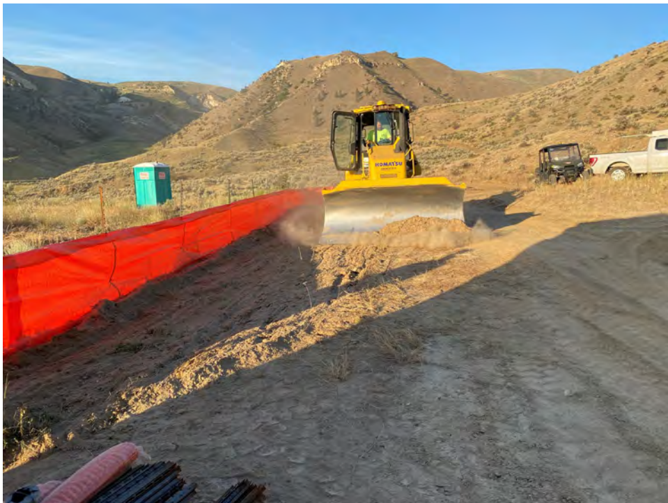
Photograph 4. Silt fence installed below soil transfer station (near SR02).
