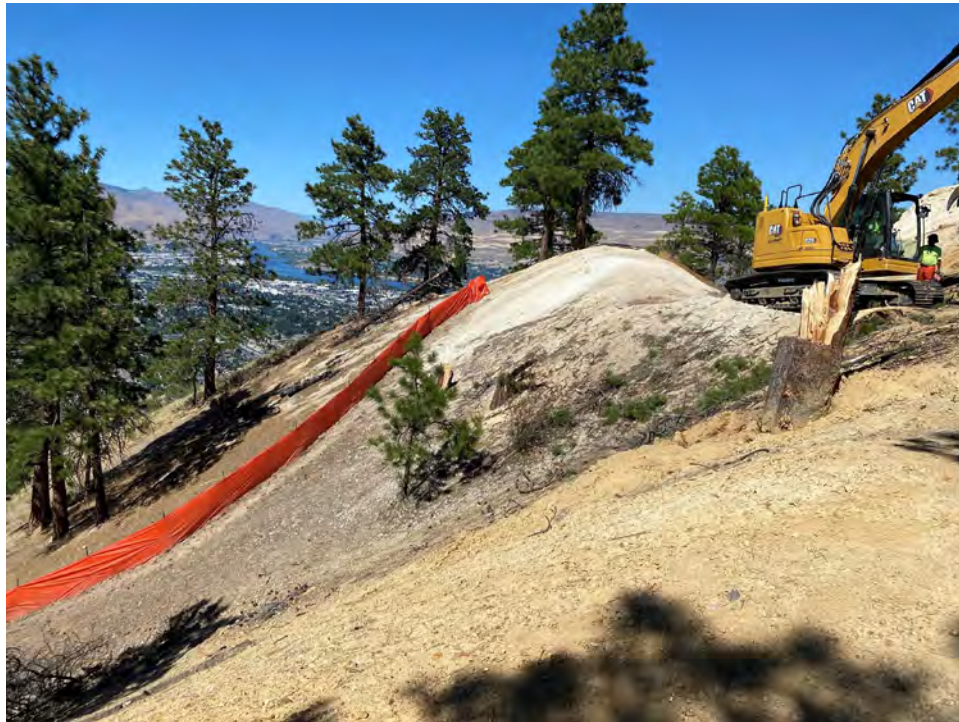
Photograph 3. Silt fence installed below SR05.
