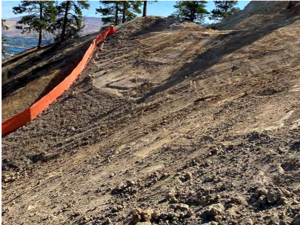
Photograph 9. Post-excavation SR05 topography (looking north).
