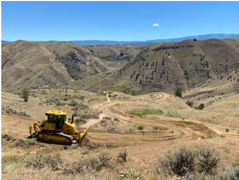
Photograph 2. Preliminary haul road improvements to provide access to SR05.
