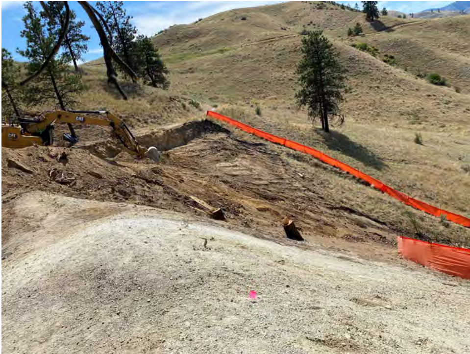
Photograph 7. SR05 waste rock and woody debris removal.
