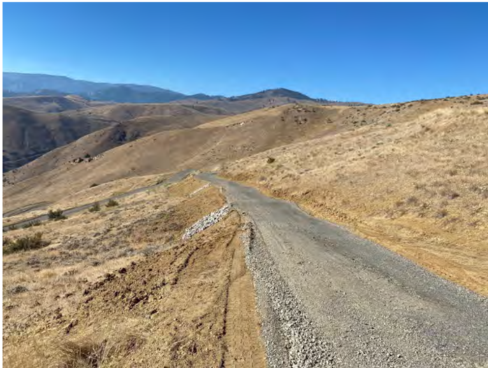
Photograph 12. Access road improvement and example stormwater features.
