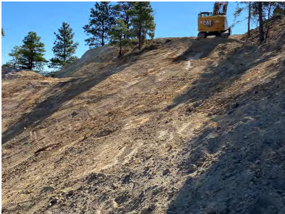
Photograph 10. Post-excavation SR05 topography (looking north).
