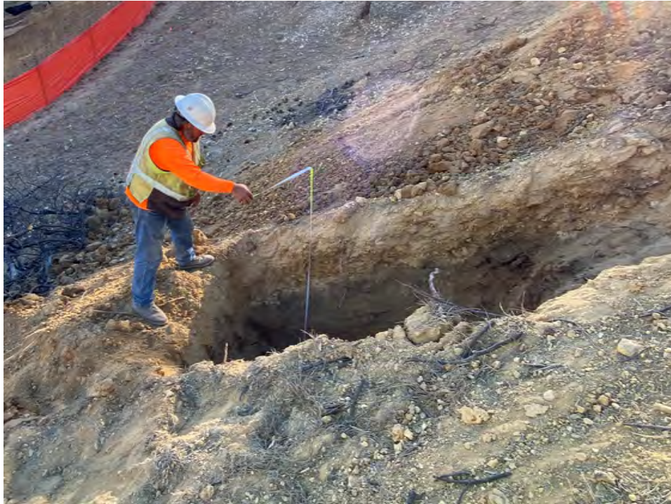
Photograph 5. Preliminary test pit exploration at SR05 (Test Pit 4).
