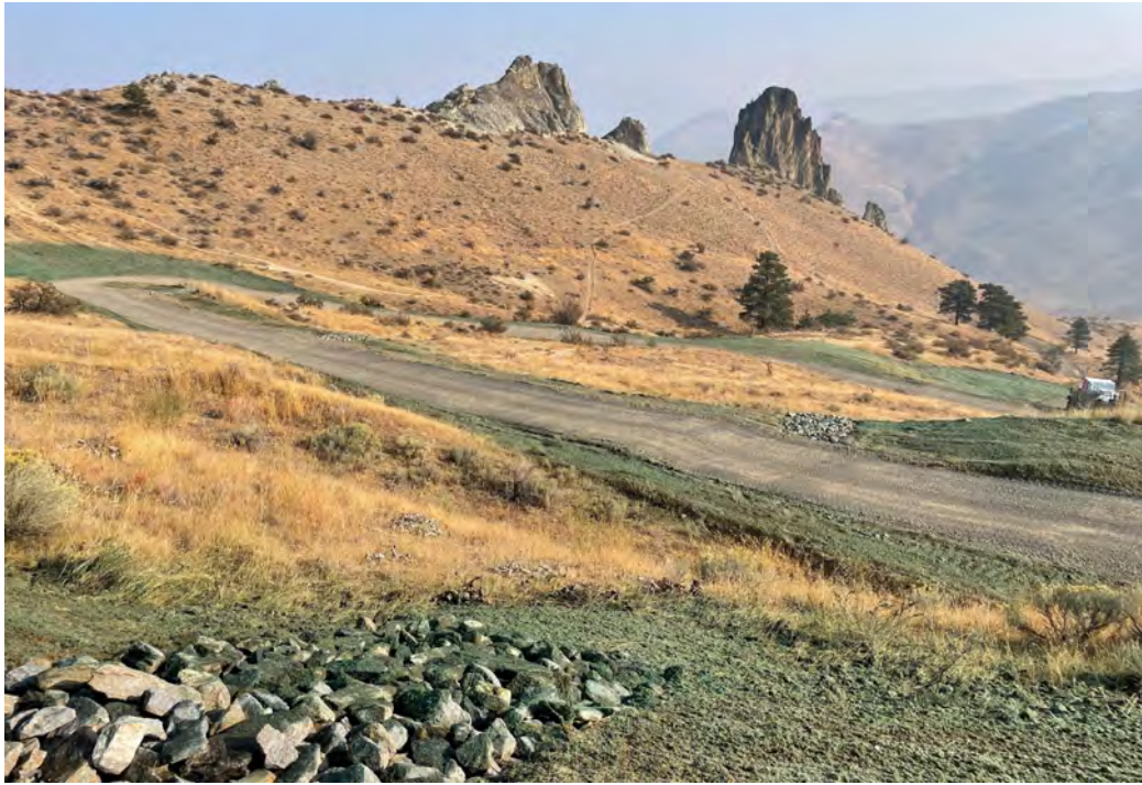
Photograph 13. Example hydroseeding activities along the upper Phase 2 haul road.
