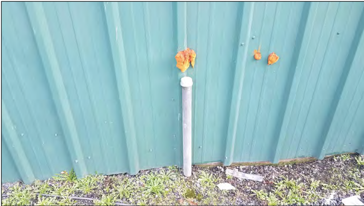
Photograph 5: Suspect UST fill port located west of the building on the central parcel at the Site.
