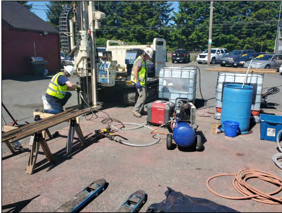
Photograph 1: View of drilling, injection tooling, air diaphragm pump, mixing tanks, rinse drums, electric compressor (later changed to gas compressor), injection manifold, generator, and various hoses and fittings. Photo taken on June 1st, 2021.
