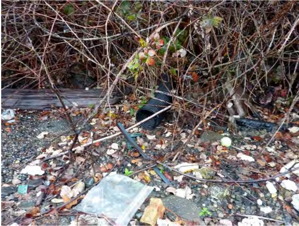
Photograph 1. Kite Hill Outfall looking north. January 1, 2010.
