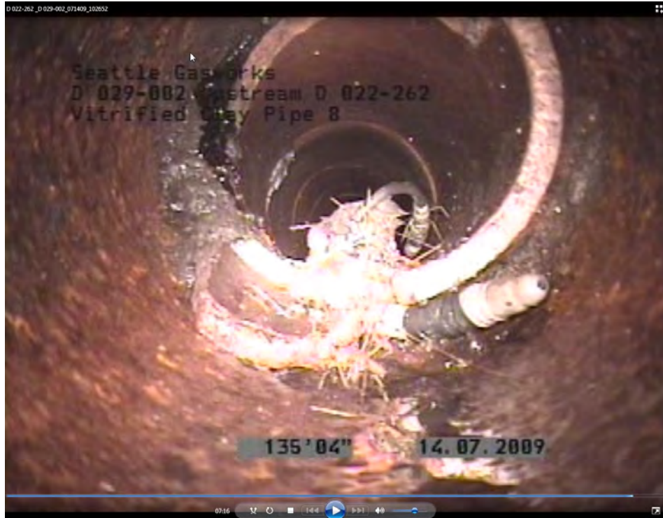
Photograph 3. SL 4 to SL 1, pipe change at 135 feet from SL 4.
