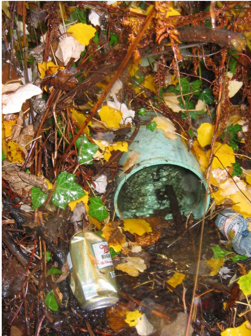
Photo 6: Waterway #19 Outfall from Culvert near Shoreline during a Storm, November 2006
