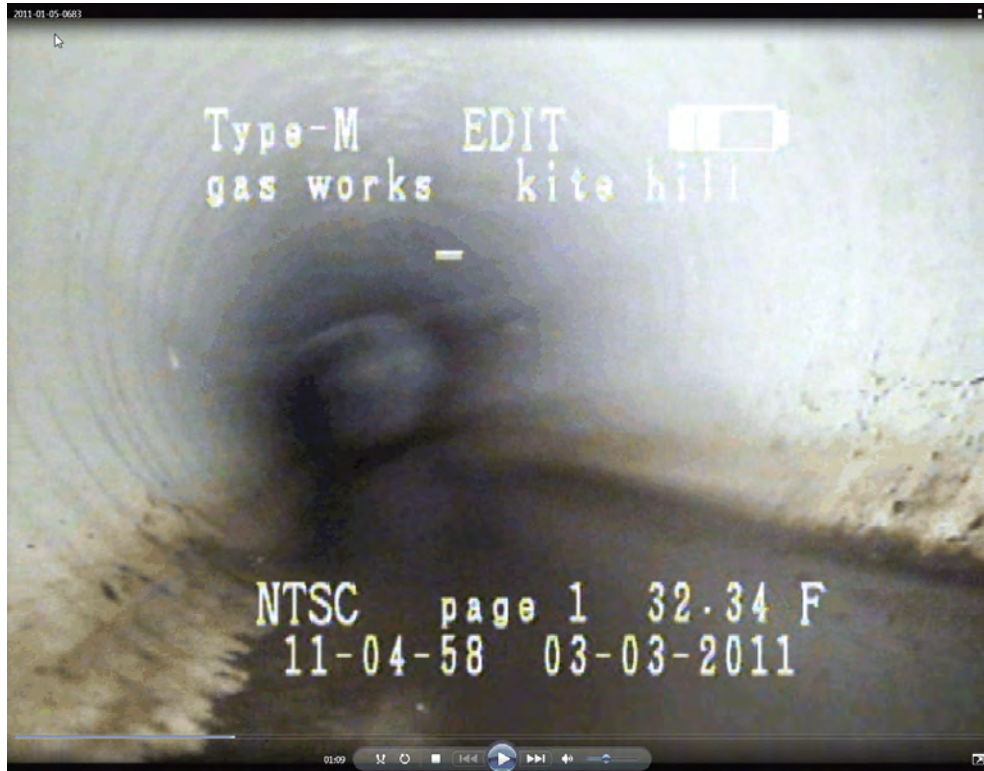
Photograph 5. Video capture of Kite Hill Manhole to Eastern Inlet. January 5, 2011.
