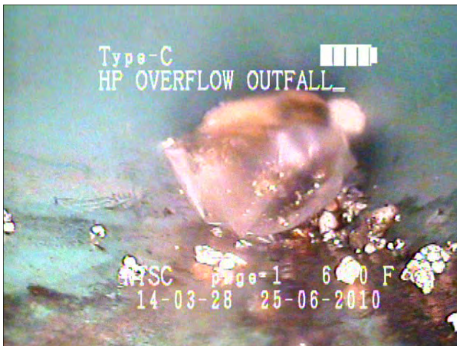
Photo: HP-CB-01_HP Over flow081359_30062010_A.jpg, VCR No.: Floyd/Gas Works 06.25.2010 5.6FT, Obstacles Other, 25 %of cross sectional area, from 04 to 08 o'clock / Plastic bag
