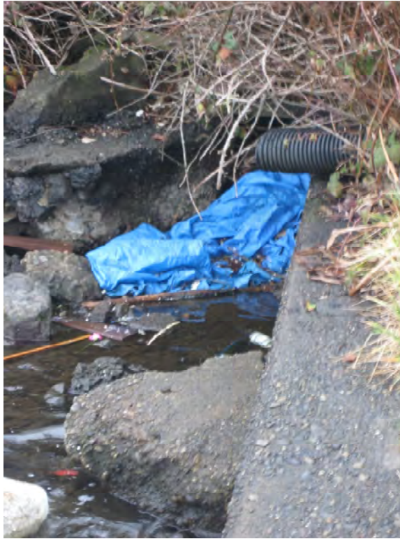
Photograph 7. Outfall F looking north. January 5, 2011.
