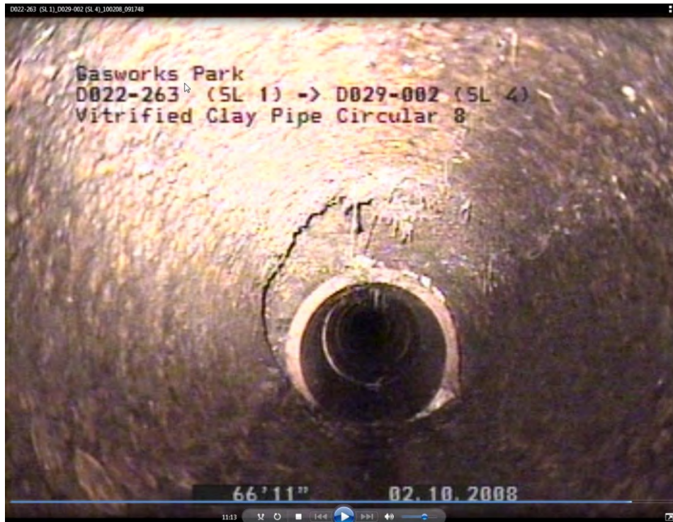
Photograph 2. SL 1 to SL 4, pipe change at 66 feet from SL 1.
