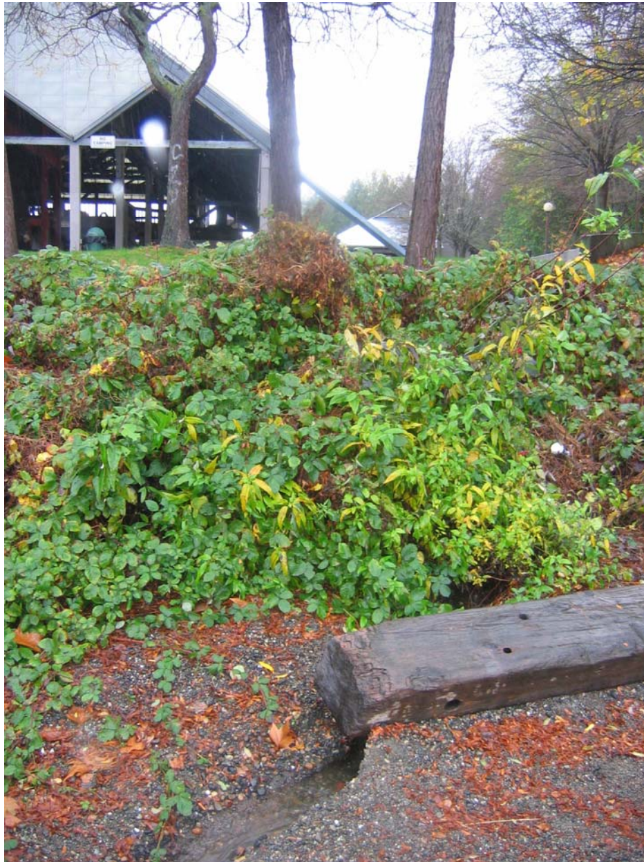
Photo 2: Discharge from Outfall B during a storm, November 2006.
