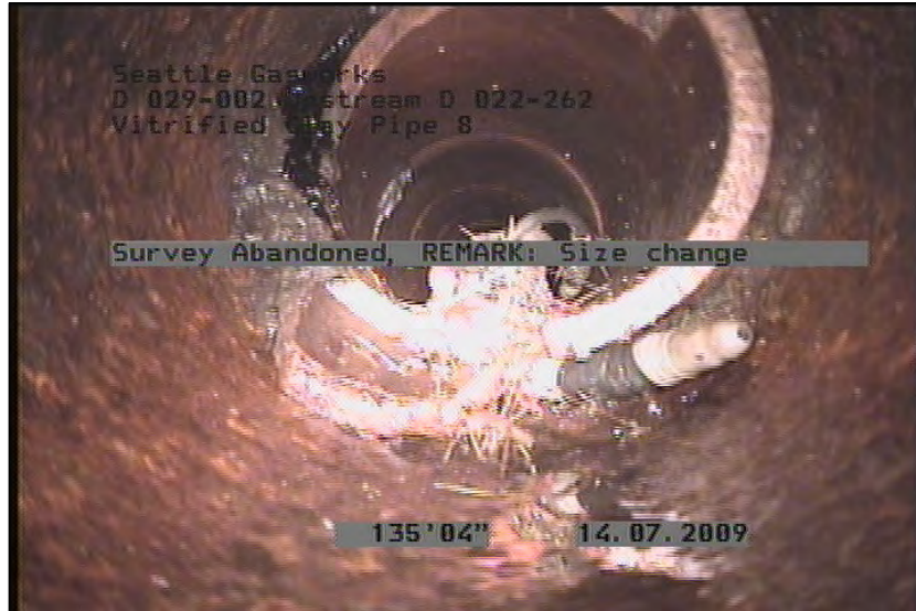
Photo: D 022-262 _D 029-002_071409_103532_A.JPG, 00:07:17 135.37FT, Survey Abandoned, REMARK: Size change
