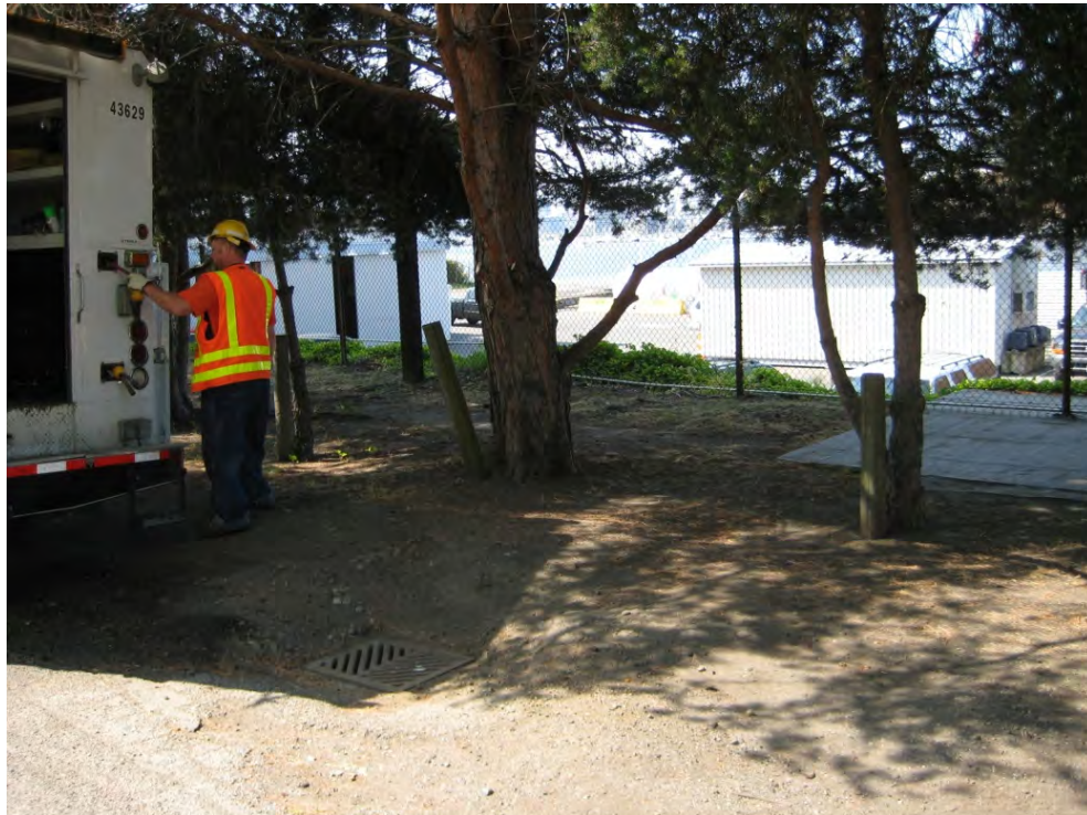
Photograph 10. Inlet on North Northlake Way.
