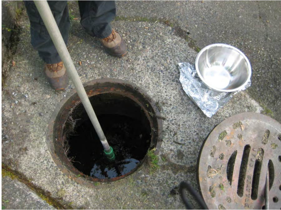
Photo 3. SPU staff sampling Catch Basin PA-CB-02 in Gas Works Park parking area.
