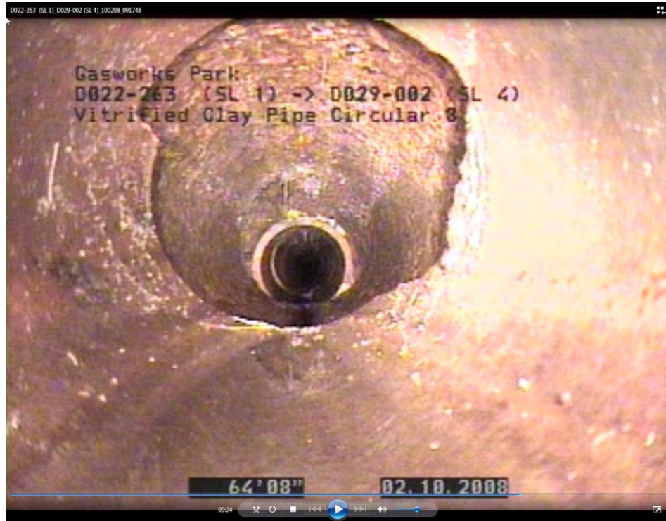
Photograph 1. SL 1 to SL 4, pipe change at 65 feet from SL 1.
