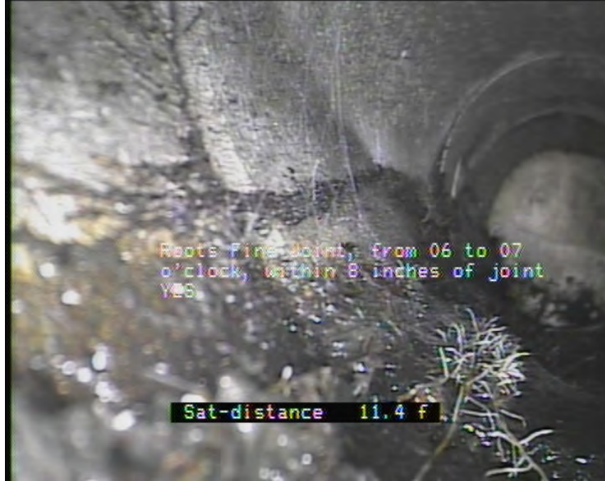
Photo: PA-CB-07_Discharge Point095728_25062010_A.JPG, VCR No.: Floyd/Gas Works 06.25.2010 11.4FT, Roots Fine Joint, from 06 to 07 o'clock, within 8 inches of joint: YES
