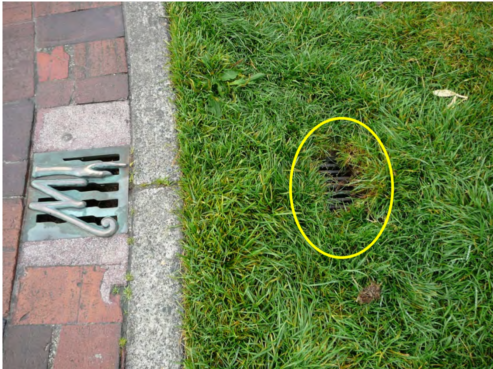
Photograph 4. Western Inlet on Kite Hill. August 22, 2011.
