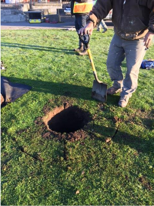
Extending sod cut
