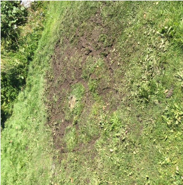
Backfilled and sod replaced Patch #1
