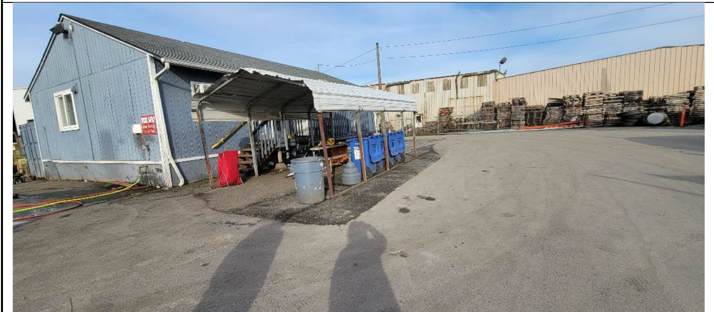
Looking southwest from near former MFG-3 well location. Older asphalt in area of lunchroom building and carport.
