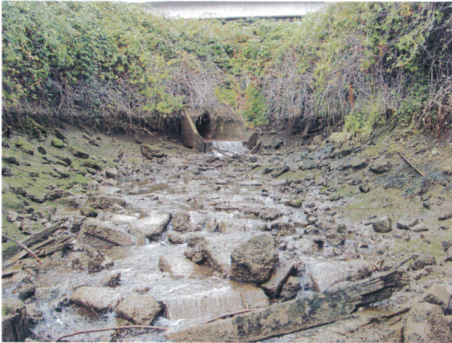
West End of Embayment (view to west toward reservoir overflow outfall)
