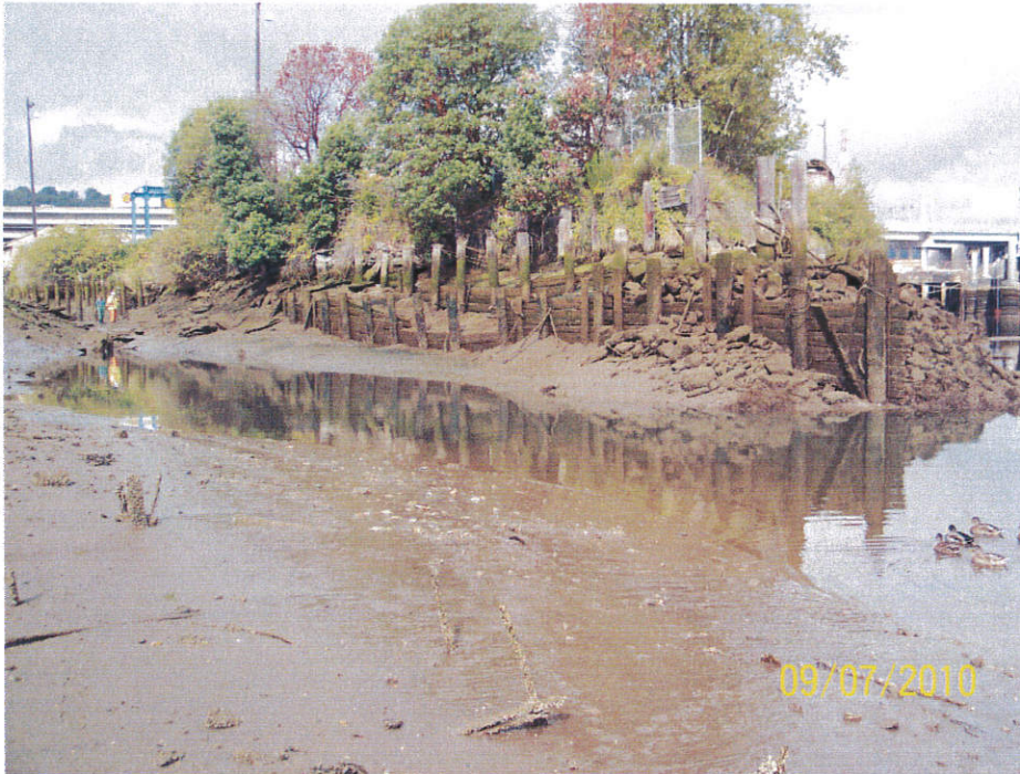
East End of North Bank (view to northwest)
