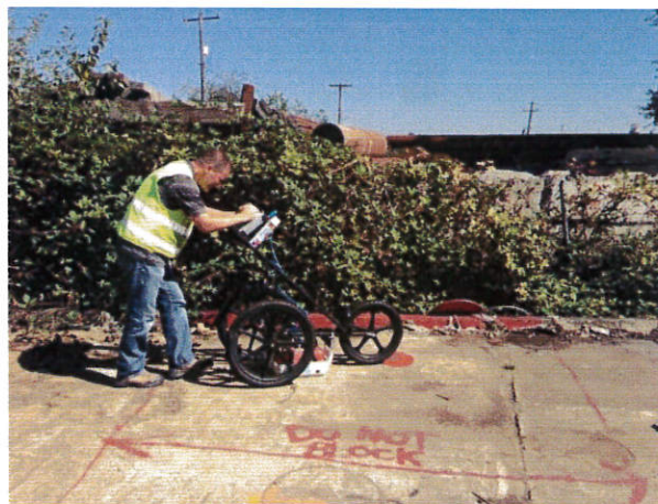
GPR survey equipment – September 9, 2013.
