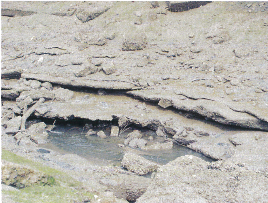
Waste Concrete Flows - North Bank - East Side of Neck (view to north)
