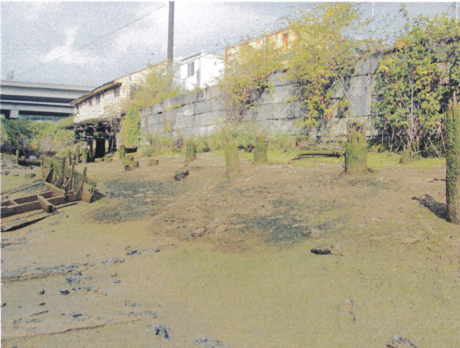
West End of North Bank (view to northwest)
