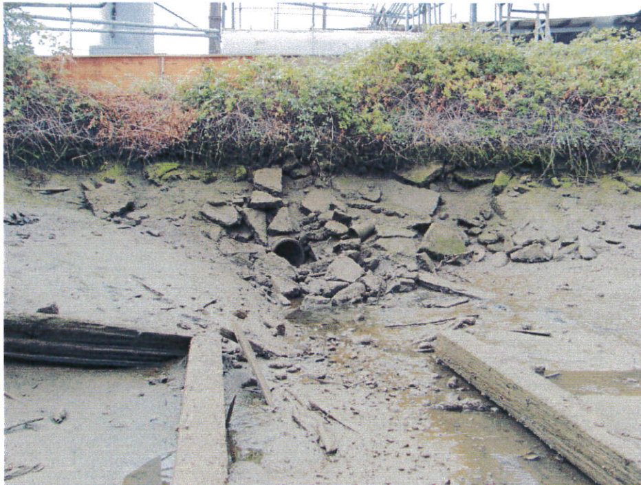
South Bank - 2nd Ave. Outfall (view to south)
