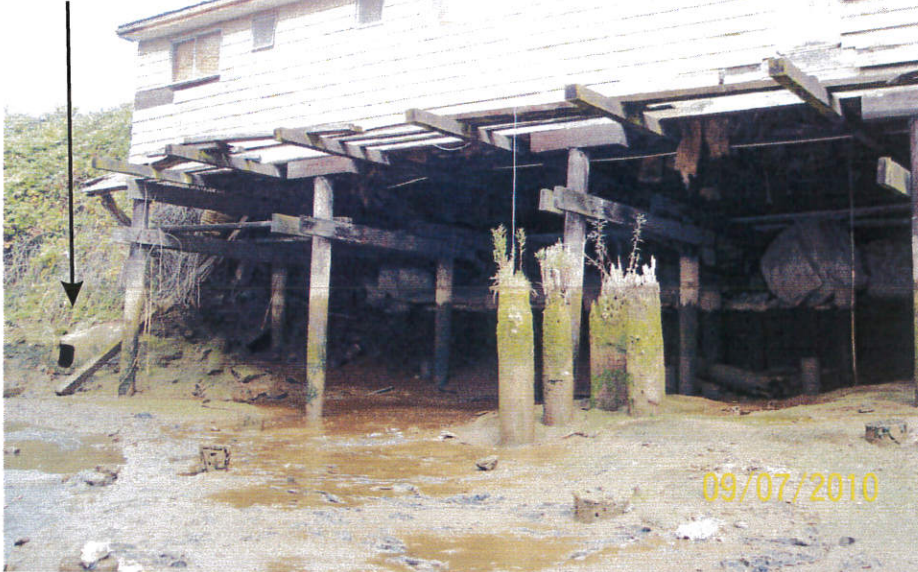
Structure West End of North Bank (view to northwest)
