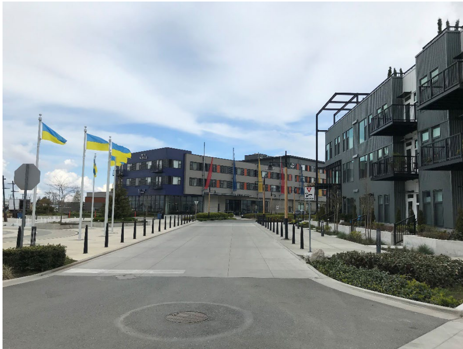
Photo 1: Southwest Corner of American Classic Homes Looking Northwest
