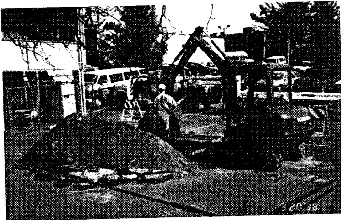
Excavation And Removal Of Diesel UST
