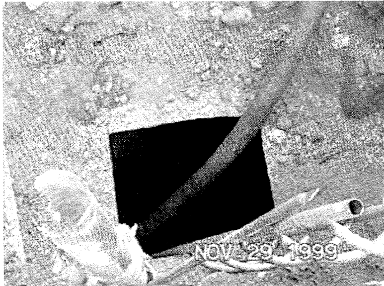
PHOTOGRAPH 2. View of access port in UST. The tank was in good overall condition.
