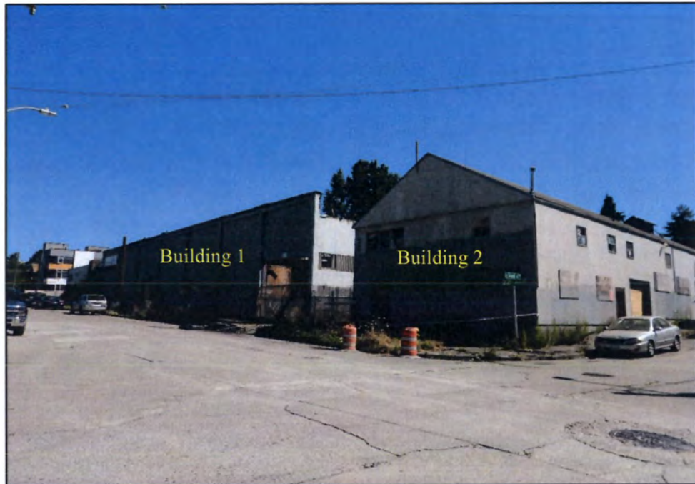
Photograph 1. Overview of the Buildings 1 and 2 exterior – Looking Northeast
