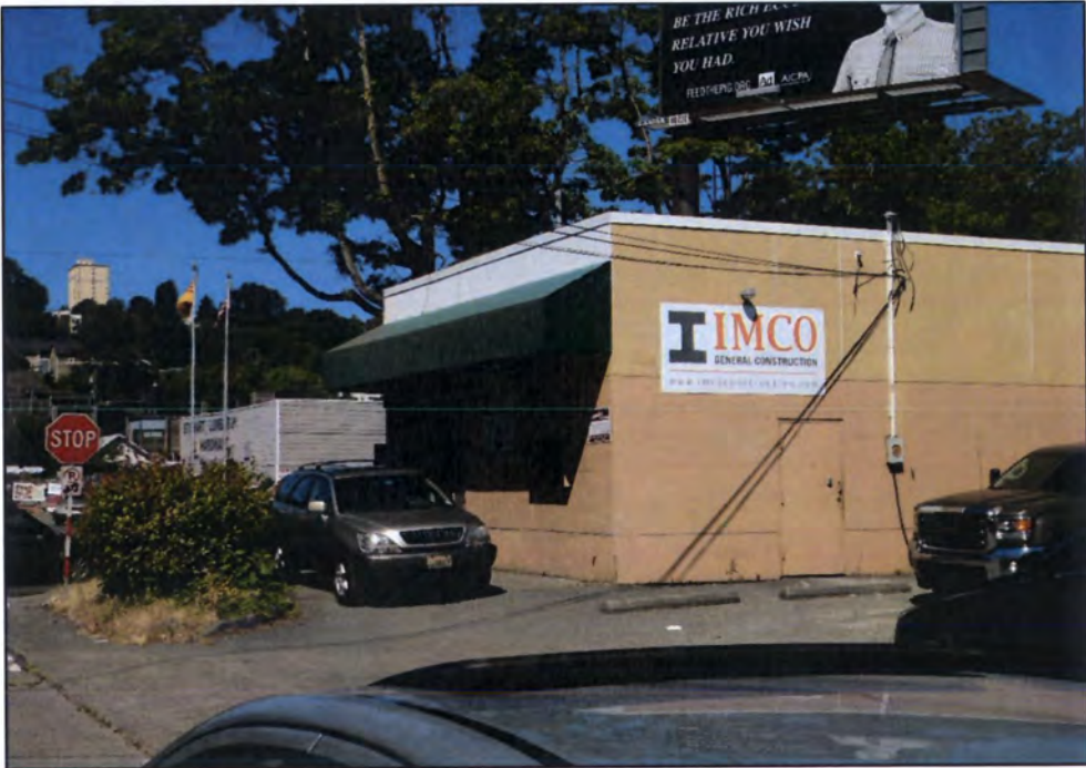
Photograph 14. Overview of the Building 4 – Looking Northwest
