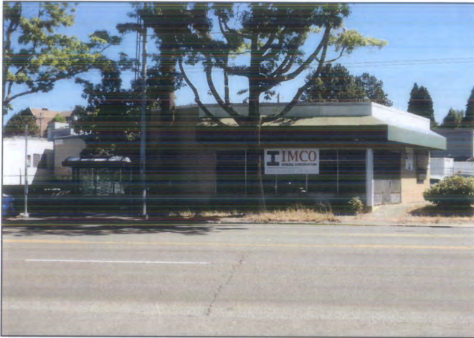
Photograph 15. Another view of the Building 4 – Looking East
