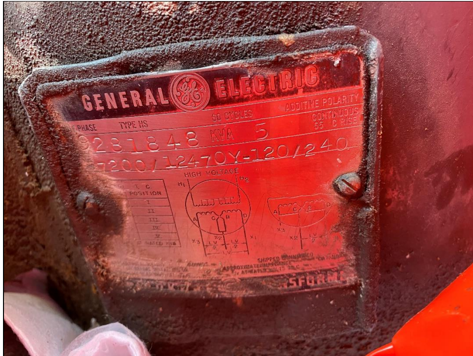
1. Transformer nameplate
