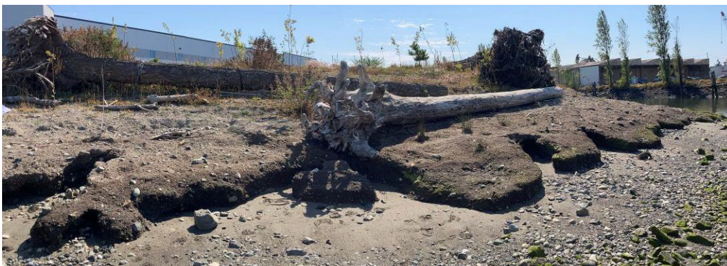
Exhibit 3-1: Southern Erosion Area on the West Shore (Photo Taken August 31, 2022)
