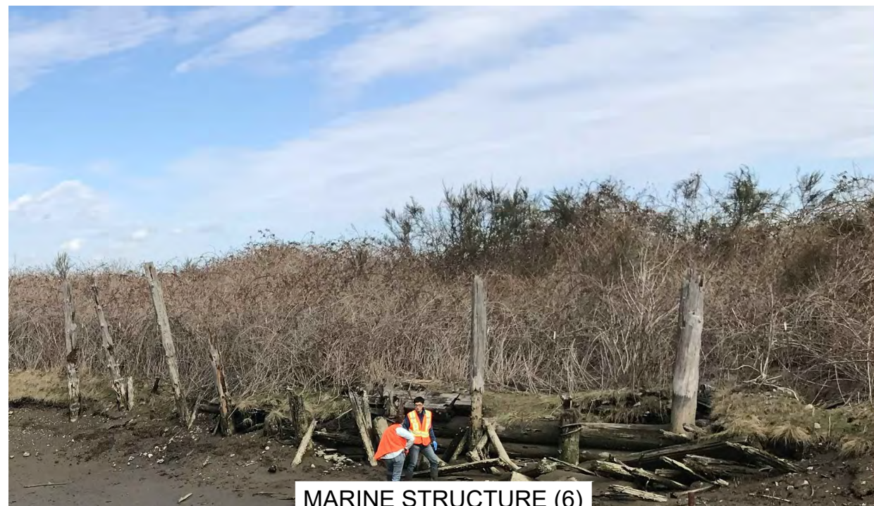
MARINE STRUCTURE (6) VIEW 1
