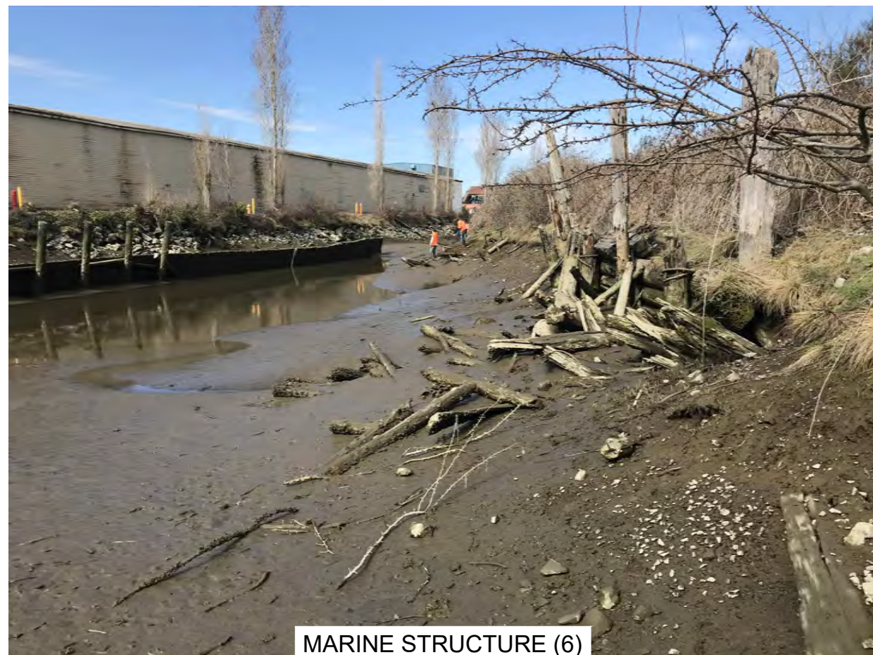
MARINE STRUCTURE (6) VIEW 2
