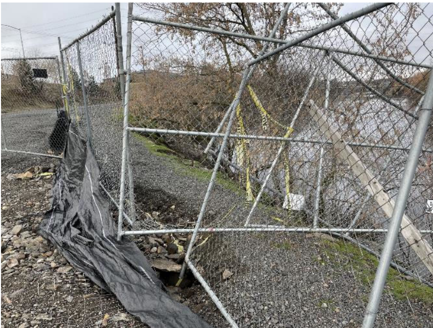
Photograph 4. Hole in temporary construction fence on the west end of the Site. Photo taken January 17, 2023.
