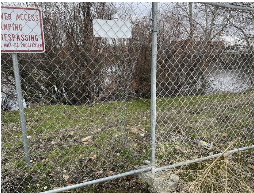
Photograph 2. Hole in temporary construction fence on the northeast portion of the Site, north of the northeast infiltration basin. Photo taken January 17, 2023.
