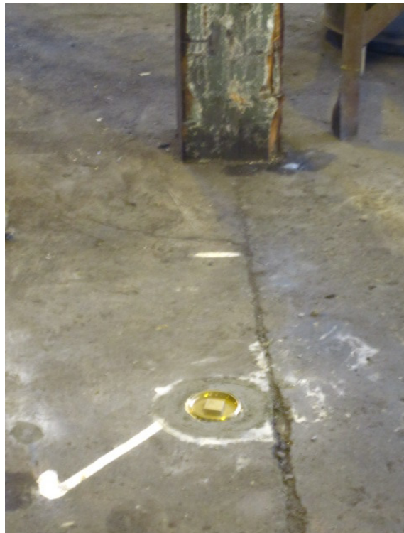
Photograph 2. Completed Vapor Point with Protective Brass Cover.
