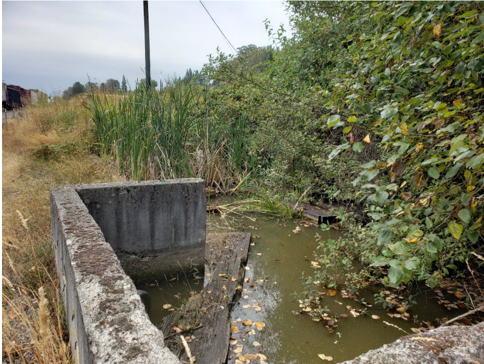
Figure 4. Artificial Feature 1 in a rectangular concrete structure.
