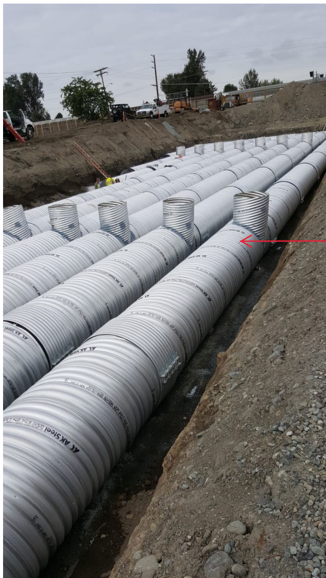
FIGURE 3 Photos of the Storm Water Detention Gallery (annotated by Ecology), October 2022. Reference: Photos provided by ECI via Email on September 9, 2022.
