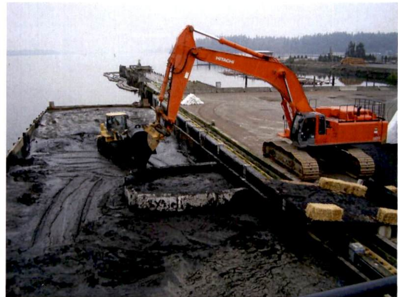
Offloading with spill plate
