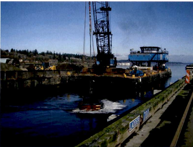
Skiff box descending for sand cover placement
