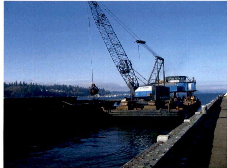
Dredge bucket offloading
