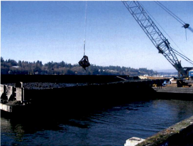
Dredge bucket offloading
