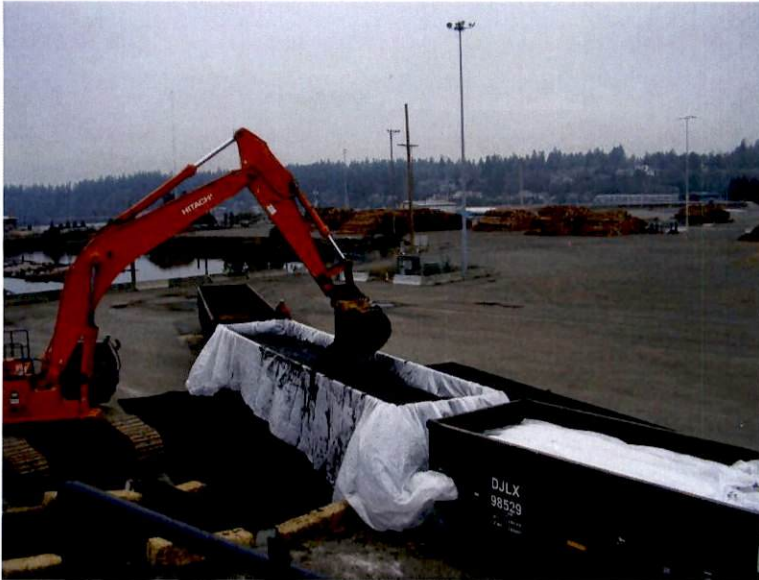
Offloading into lined railcar
