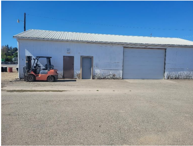
Photo 1. View of northeast side of warehouse building facing southwest. Photo taken on 5/11/2022.
