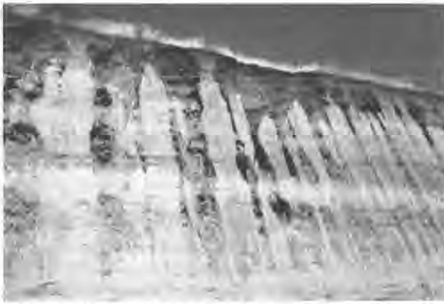
FIGURE 14 Erosion and piping damage in near-vertical cut in loess.
