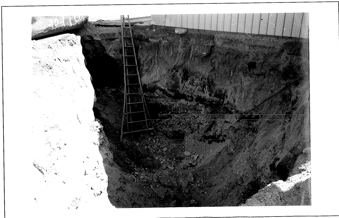
VIEW INTO THE EXCAVATION SHOWING THE SILTY SAND OVERLAYING THE GRAVEL.
