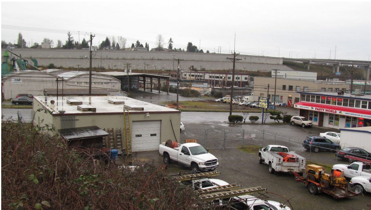
Photo 2: North Side of Facility - from the north
