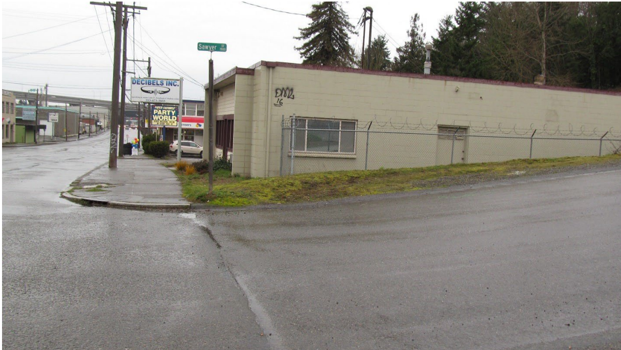
Photo 1: Former Alpine Plating Facility – from the east
