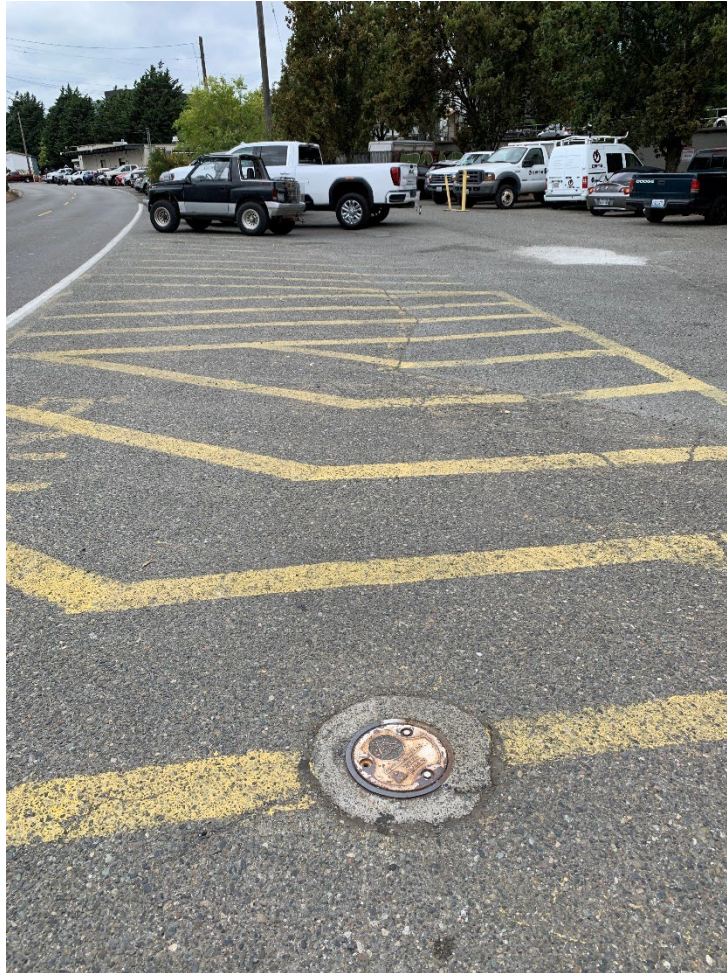
Photo 9: Monitoring well and pavement within the right-of-way area.
