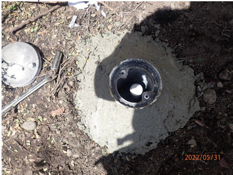
EMW01 was completed as a permanent monitoring well with 1.25-inch PVC casing and 10 feet of well screen from 9.5 ft to 19.5 ft.
