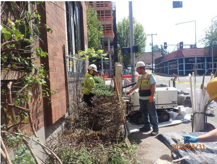
EMW01 was moved 2 feet north after encountering a PVC pipe at the first location.
