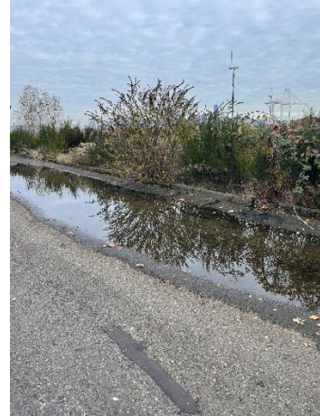
Photo 4: Ponding water (Figure 1, Note 6).
