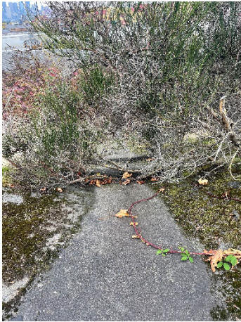
Photo 1: Vegetation overgrowth obstructing drainage swale (Figure 1, Note 3).
