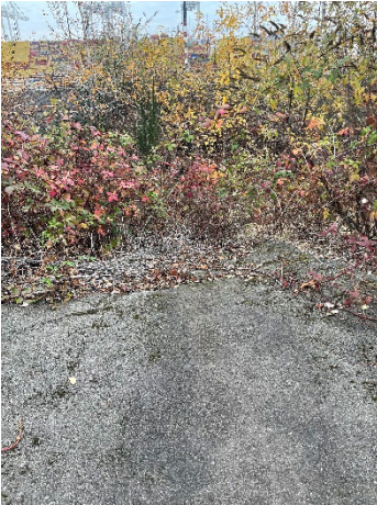
Photo 3: Vegetation overgrowth obstructing drainage swale (Figure 1, Note 5).
