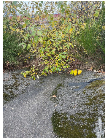
Photo 2: Vegetation overgrowth obstructing drainage swale (Figure 1, Note 4).
