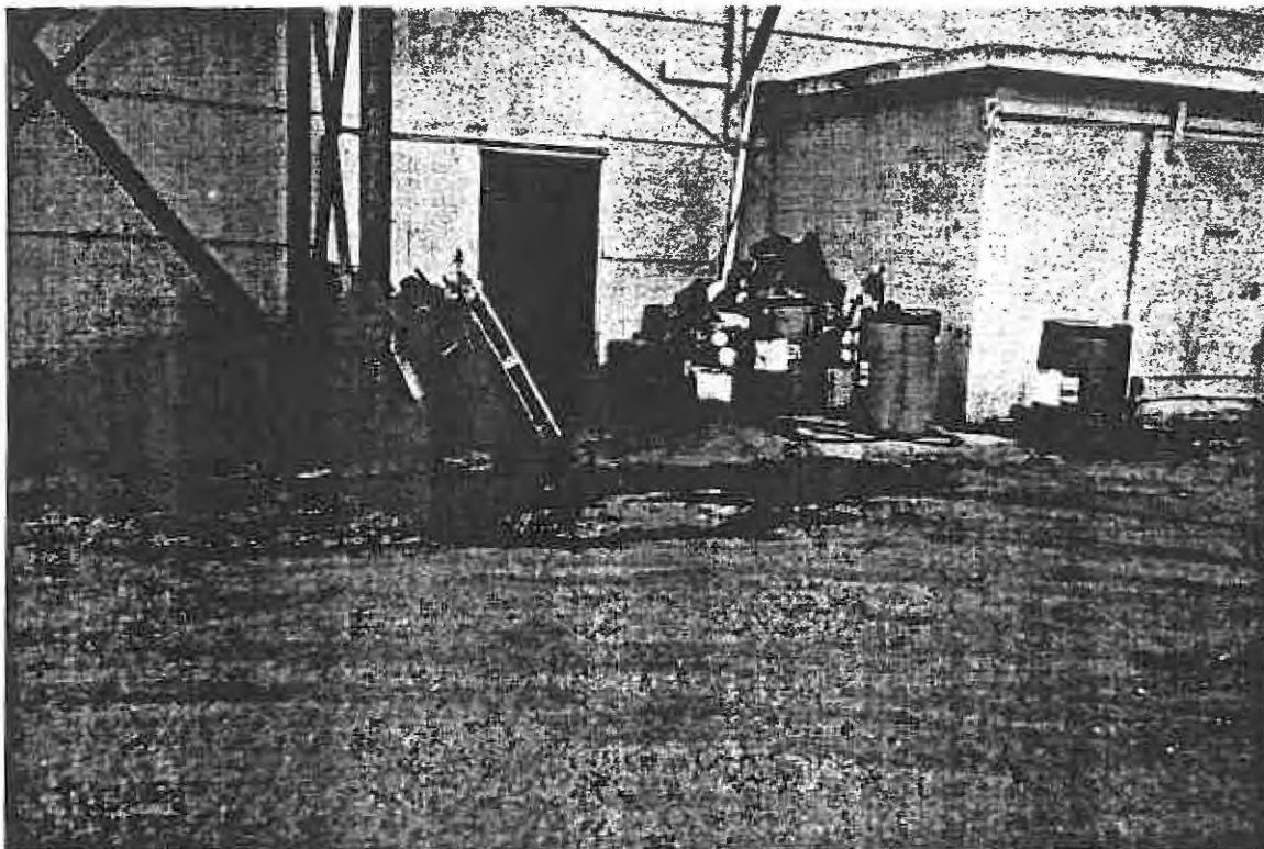
23 Overview of west entrance to planer building and stained soil (SS-1)
