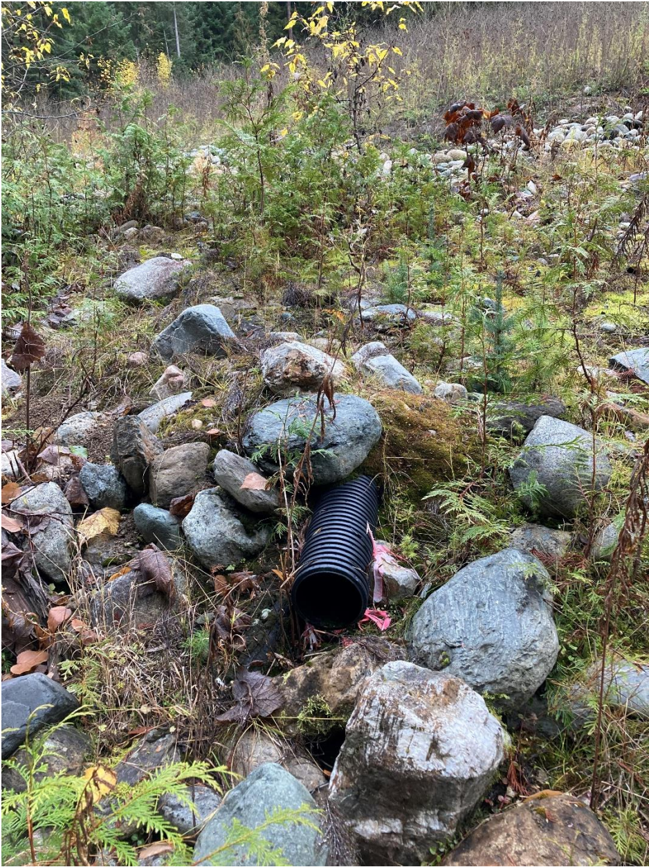
Photo 4: French drain output, looking northwest along northern edge of capped area
