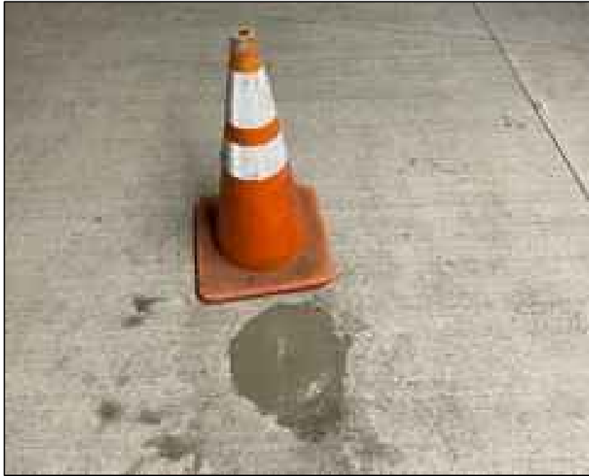
Photograph 11: Photo of well RW-2 after decommissioning was completed.
