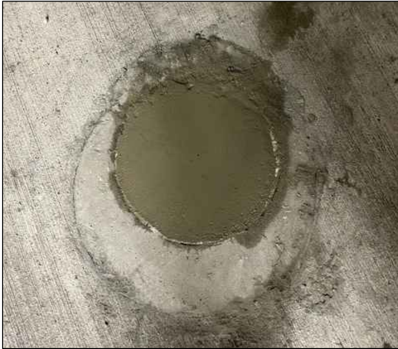
Photograph 7: Photo of well MW-6 after decommissioning was completed.
