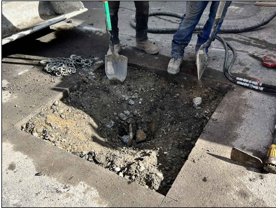
Photograph 3: View of well MW-5 location after well monument was removed.
