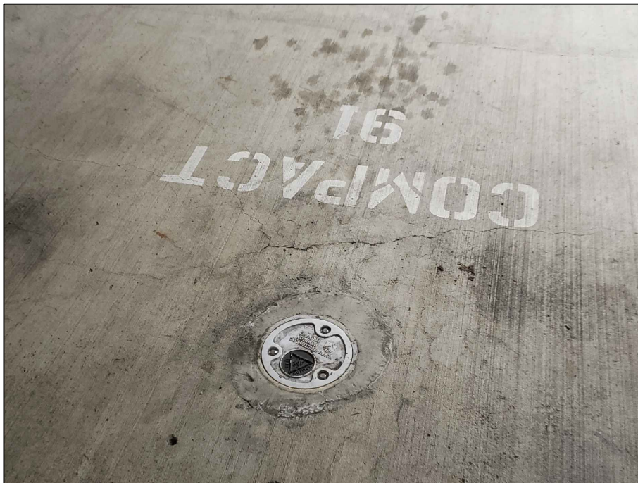
Photograph 6: Photo of well MW-6 facing northwest in the parking garage prior to decommissioning.
